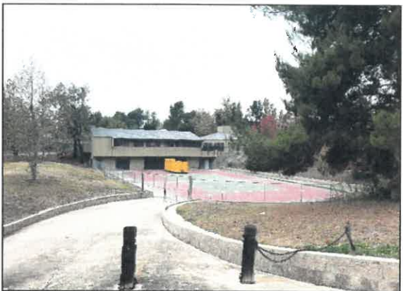
6. View looking north from the southern end of the property.
