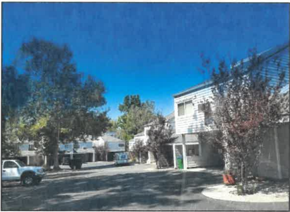
8. View of Village Condominiums.
