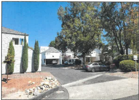
11. View of Village Condominiums.
