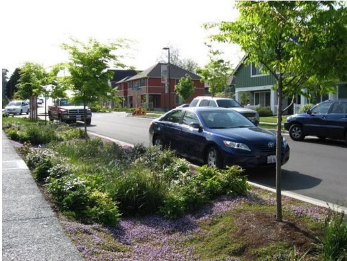
**Figure 1. The street-side swale and adjacent porous concrete sidewalk are located in the High Point neighborhood of Seattle, WA**
