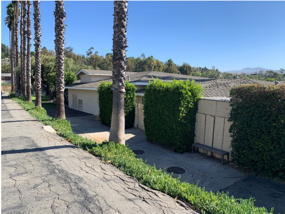
Figure 5-4 Clubhouse, northwest elevation, facing south
