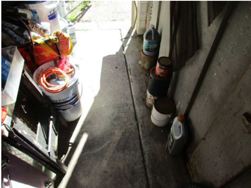
Photo 10 – Paints and lubricants adjacent to transformer cage.
