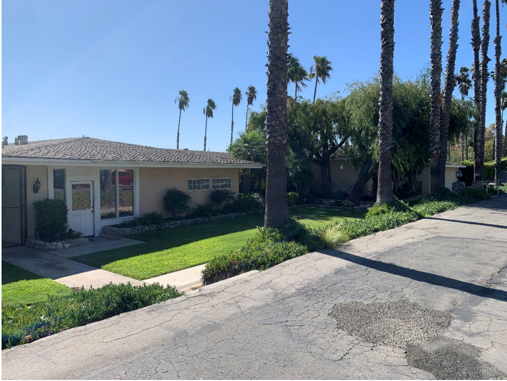
Figure 5-3 Clubhouse, northwest elevation, facing south
