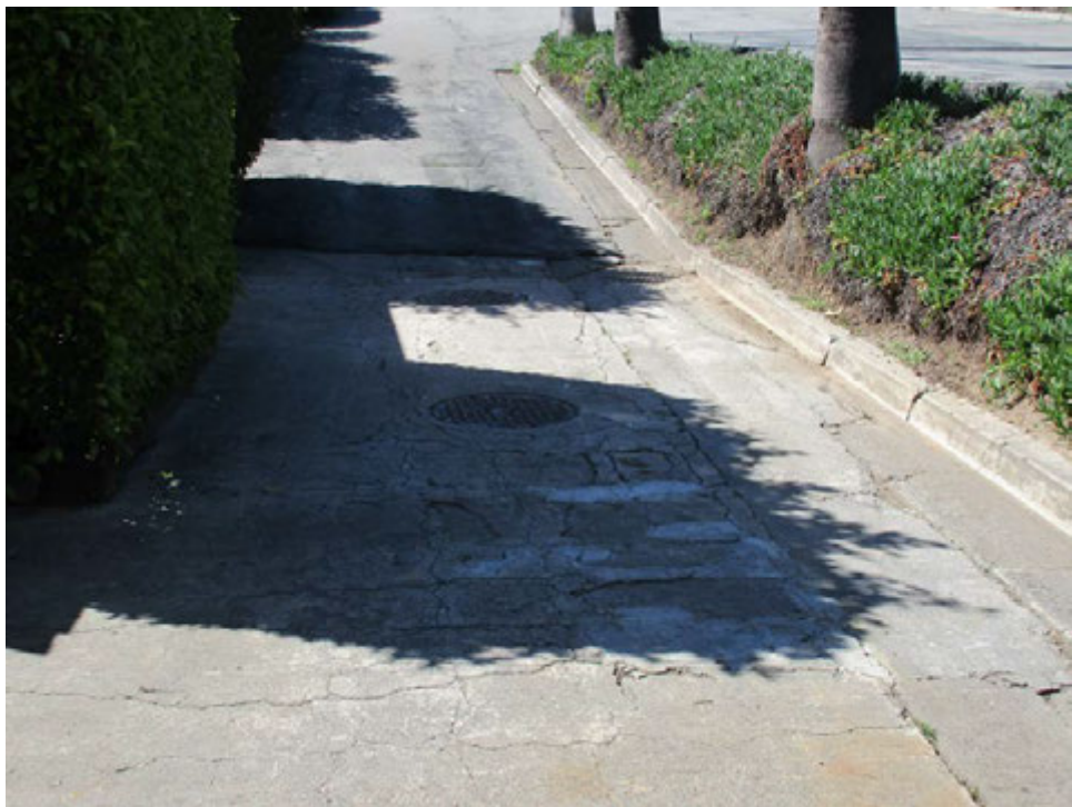
Photo 12 – Sewer manhole covers southwest of the clubhouse.
