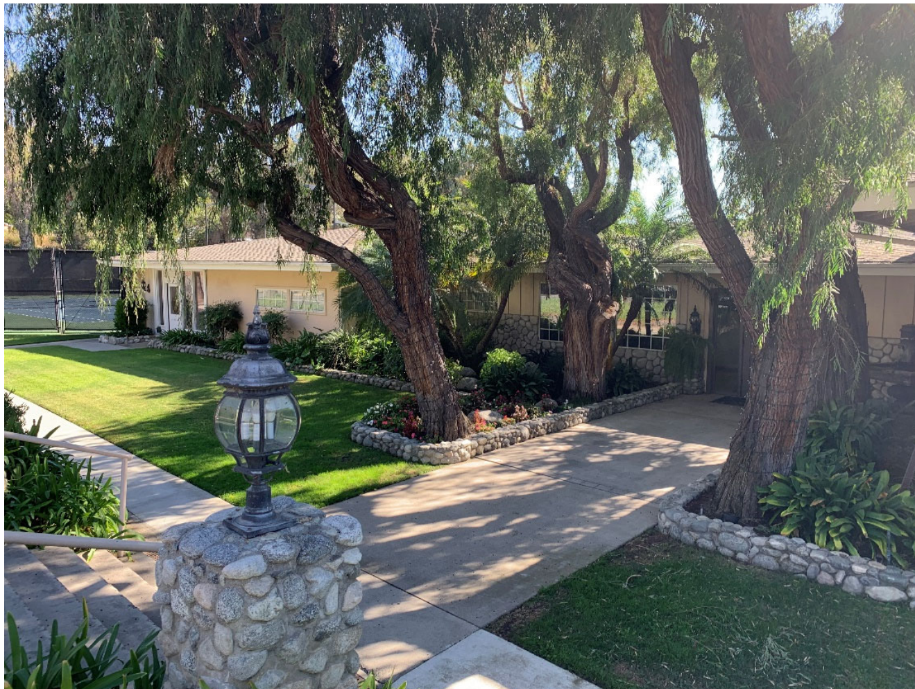
Clubhouse, northwest elevation, facing north
