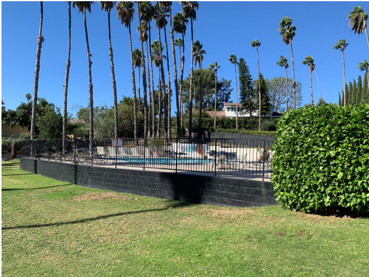
Swimming Pool, facing west
