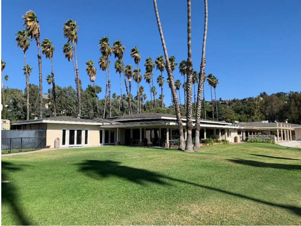
Figure 5-1 Clubhouse, southeast elevation, facing north
