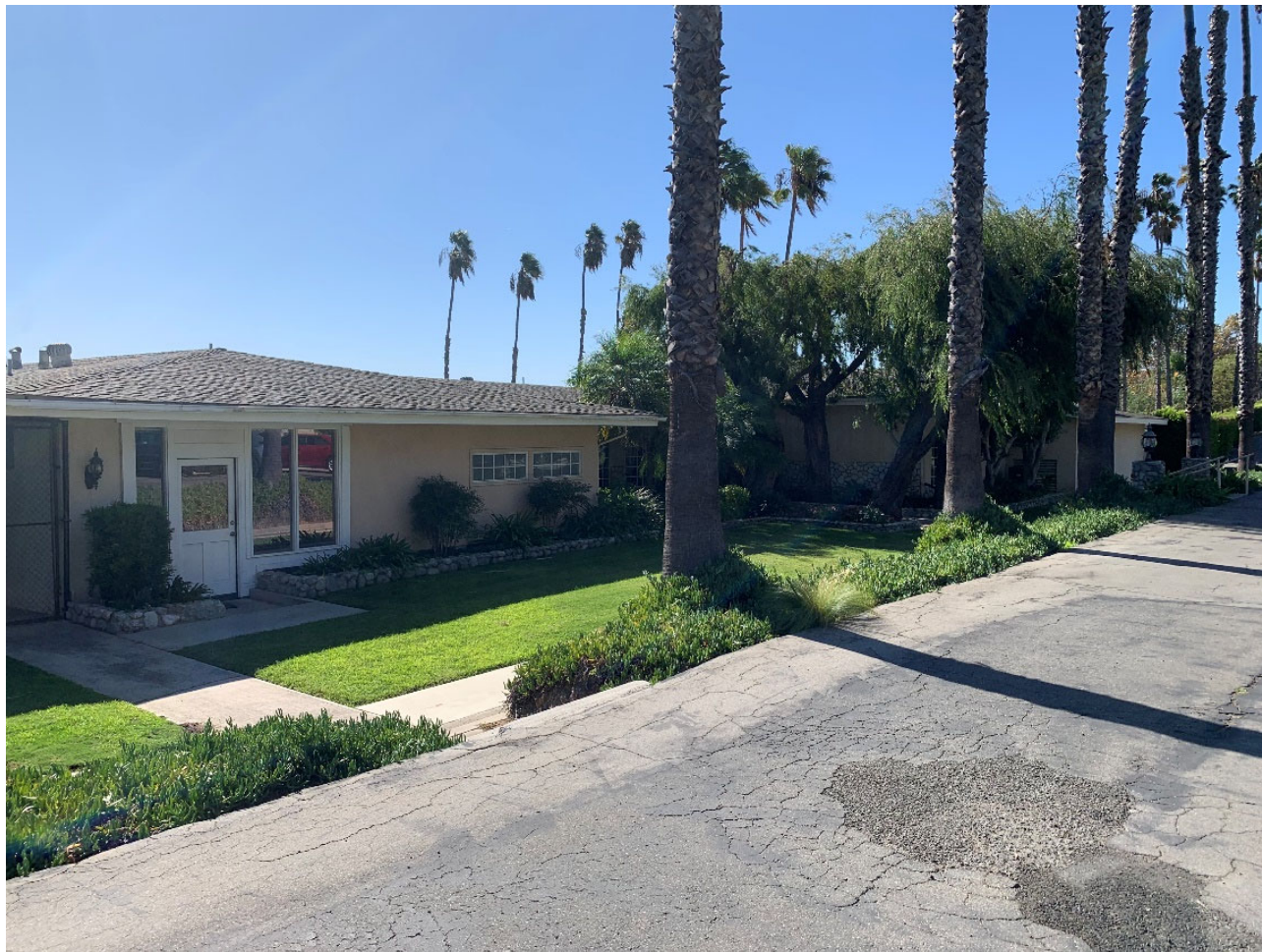
Clubhouse, northwest elevation, facing south
