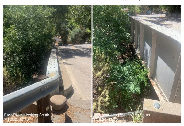
Photo 9. East side of the Bridge, looking south; treated wood posts and peeling yellow paint along guard rail.
