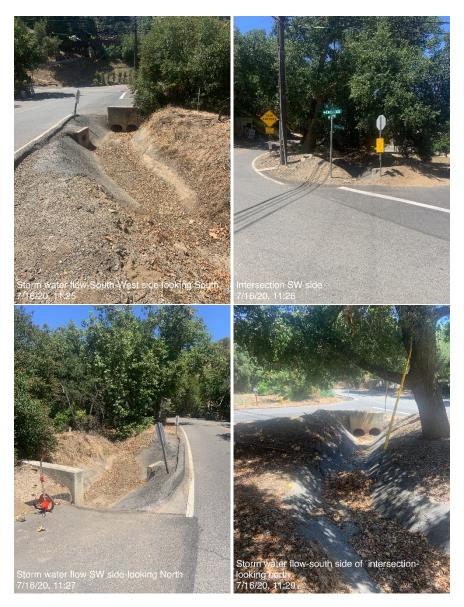
Photo 11. Southwest side of the Bridge; stormwater flows through concrete-lined culverts and ditches.
