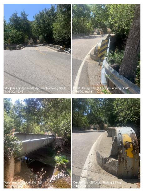
Photo 1. Modjeska Canyon Road Bridge (No. 55C0172) (Bridge), looking south over Santiago Creek, a utility pipe runs parallel to the west railing; metal guard rail is rusted with peeling yellow paint and damaged concrete curb. Concrete and asphalt along this Bridge are weathered.
