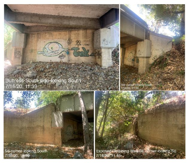
Photo 14. South side of the Bridge, looking south (top left), southeast (bottom left), and southwest (top right); the retaining wall at the southeast corner is exposed (bottom right).
