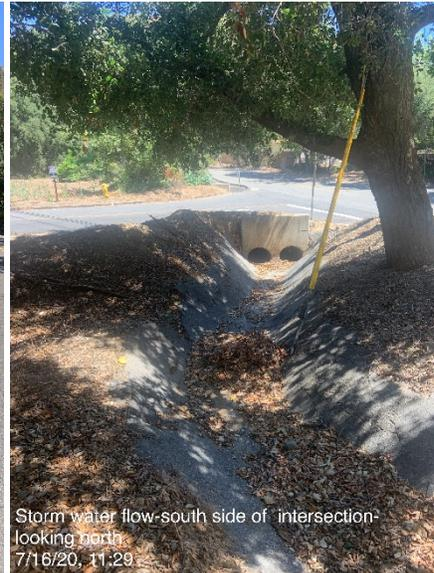
*Photo 11. Southwest side of the Bridge; stormwater flows through concrete-lined culverts and ditches.*
