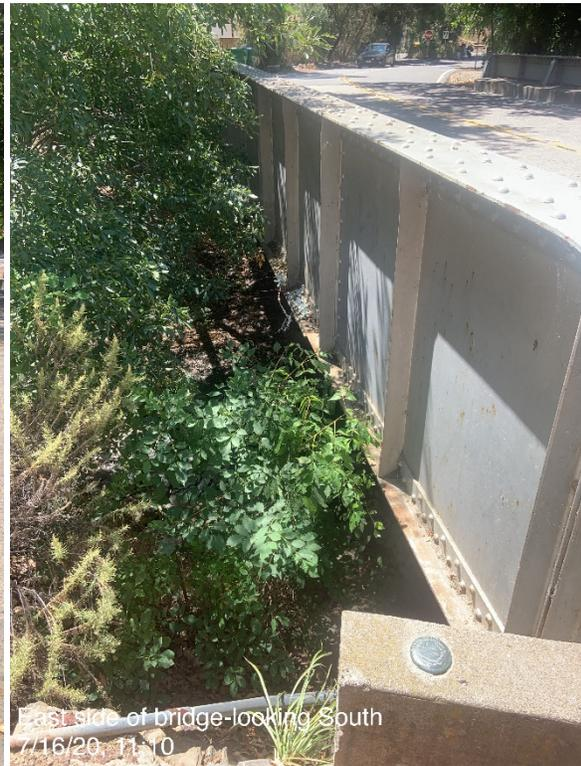
*Photo 9. East side of the Bridge, looking south; treated wood posts and peeling yellow paint along guard rail.*
