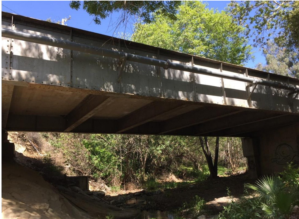
Facing east (upstream)
