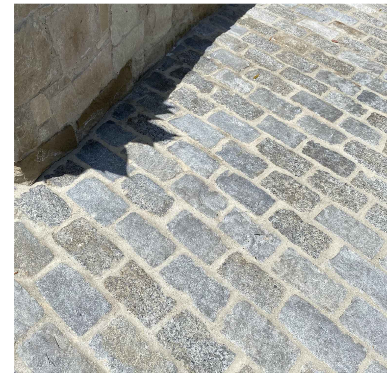
COBBLESTONE DRIVEWAY PAVING
