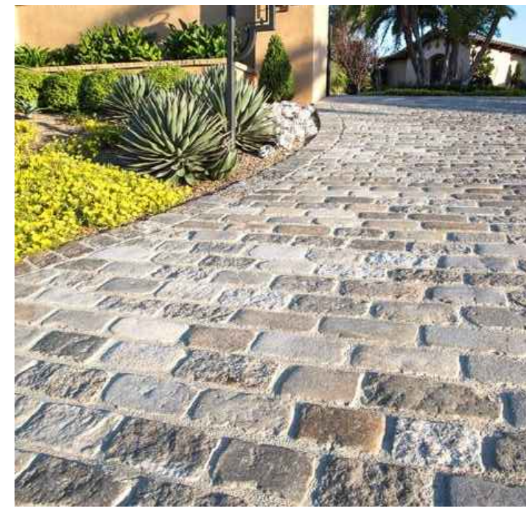
COBBLESTONE DRIVEWAY PAVING
