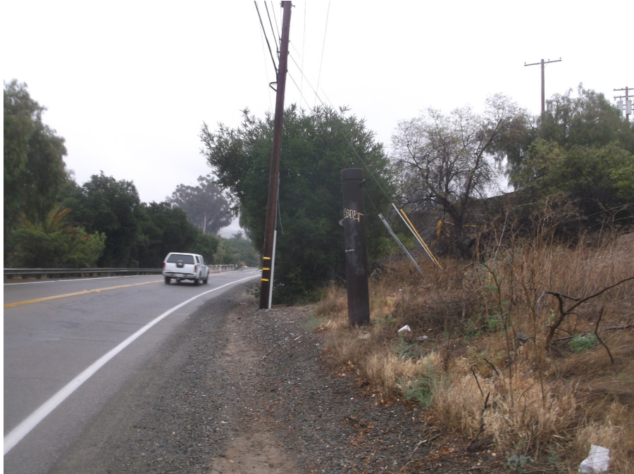
Plate 25: Jackline Support (Center), View Northeast.
