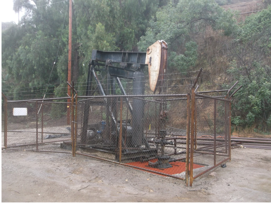
Plate 24: Brea Well #80, View Southeast.
