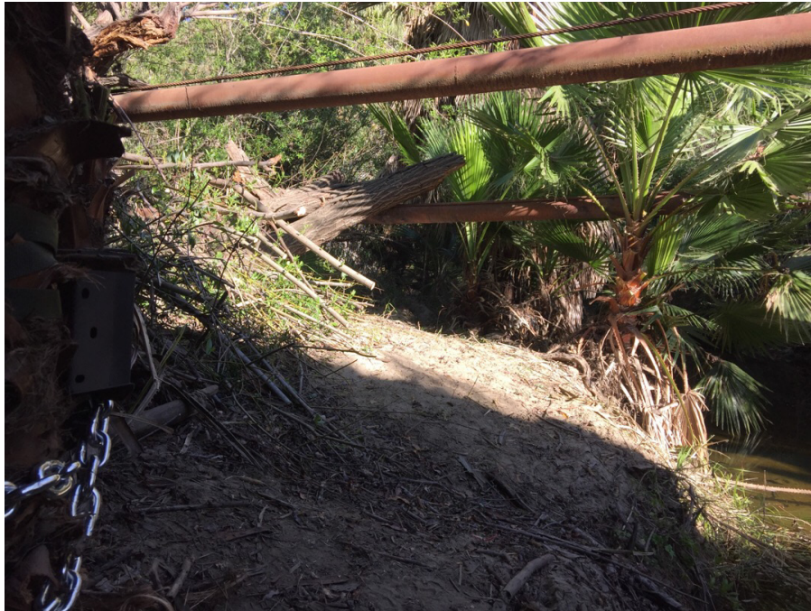
Photograph 5: View east from Camera 3 of wildlife trail along the north side of the north span underneath Bridge 1.
