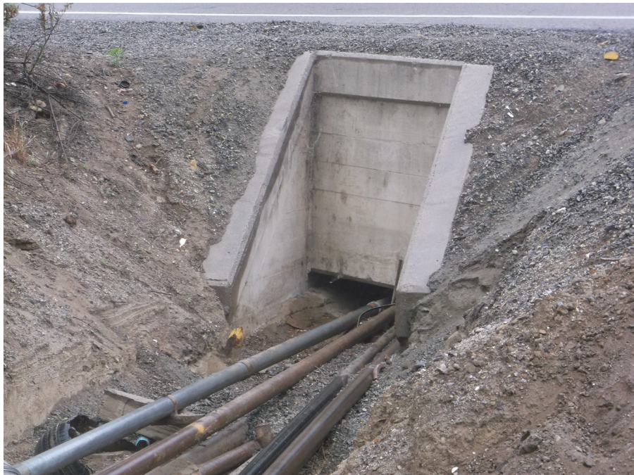
Plate 5: Oil Line Culvert.
