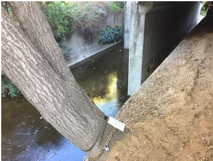
Photograph 12: View southeast from Camera 10 looking under Bridge 3 at Brea Creek. Bridge 3 has three spans and Camera 10 was angled to capture wildlife moving through the eastern-most bridge spans.
