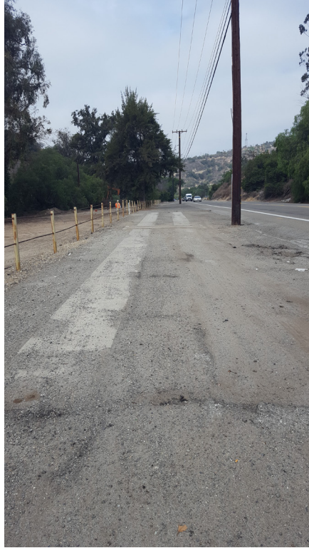
Plate 7: Abandoned Weigh Station, View West.
