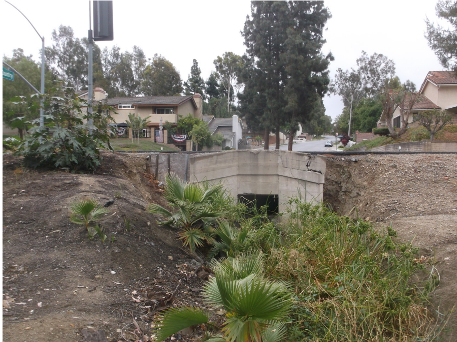
Plate 4: Drainage Culvert at Canyon Country Road.
