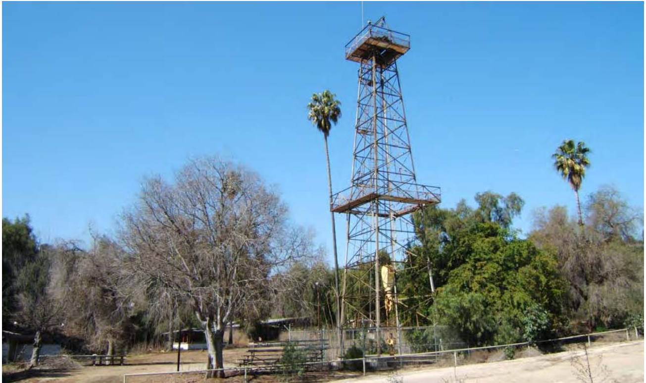
P5b4. UNOCAL employees' park, facing WNW, 22 February 2006. 1927 "Stearns 71" derrick preserved amid steel events shed (middle distance), wood kiosk (left of bare tree in foreground), and concrete-block restrooms (far left in trees).
