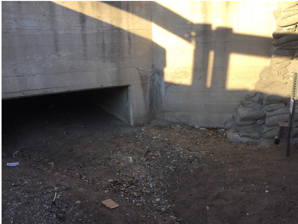
Photograph 14: View of Camera 12 (located on the south side of Brea Boulevard) pointed northwest and looking into Culvert 2.
