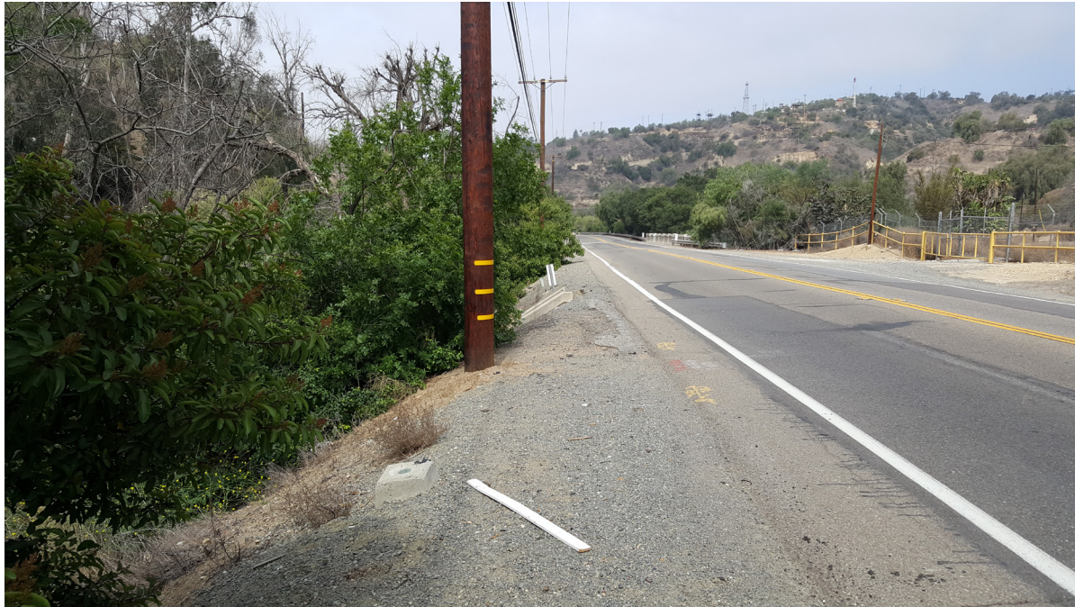
Plate 3: Brea Boulevard East of Bridge #55C0123, View West. Note Culvert and Geodetic Benchmark on Shoulder.
