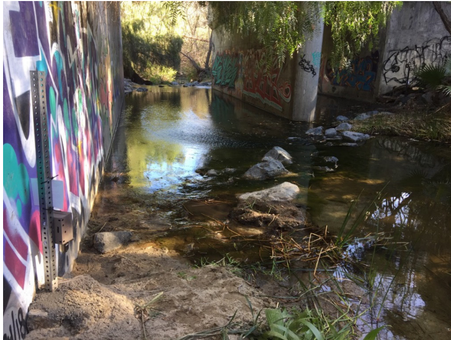
Photograph 7: View south from Camera 5 (located on the west side underneath Bridge 2) that shows both spans of Bridge 2, with Brea Creek flowing south through both bridge spans.
