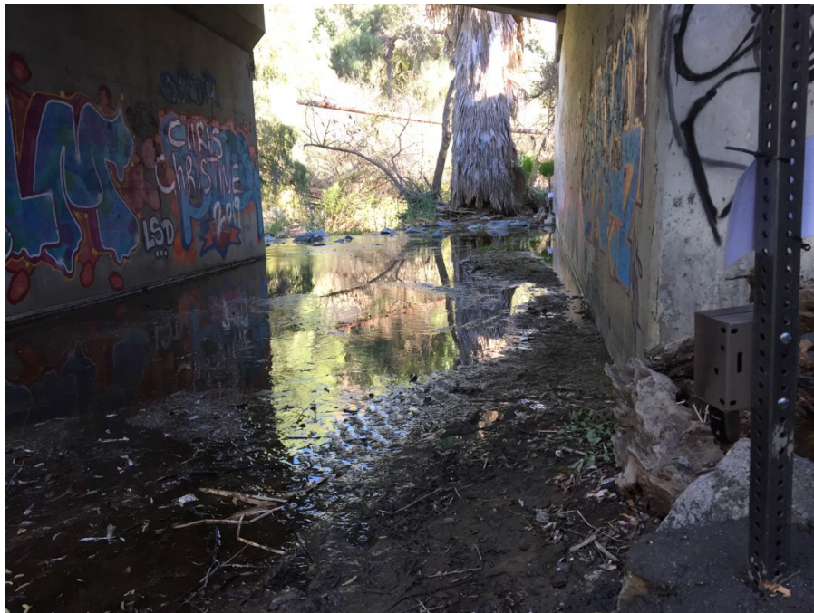
Photograph 6: View southeast from Camera 4 (located on the west side underneath Bridge 2) looking underneath the south span of Bridge 2. Brea Creek flows south through Bridge 2, but is relatively shallow (less than a foot deep) with a cement, rock, and sandy bottom.
