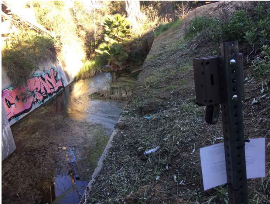
Photograph 11: View southeast across Brea Creek from Camera 9 (located on the west side of Brea Creek and Bridge 3 and the south side of Brea Boulevard).
