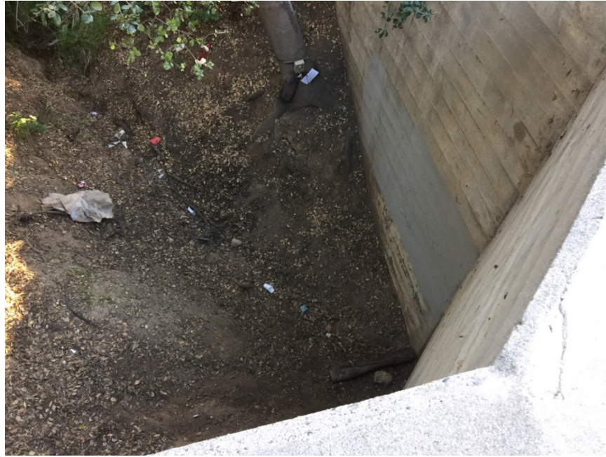
Photograph 15: Top-down view of Camera 13 (attached on a Coast live oak tree on the south side of Brea Boulevard) which was angled north looking into Culvert 3.
