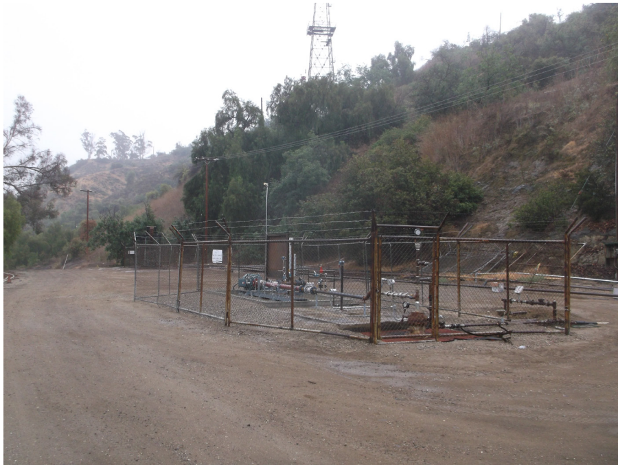
Plate 21: Brea Well #53, View East.
