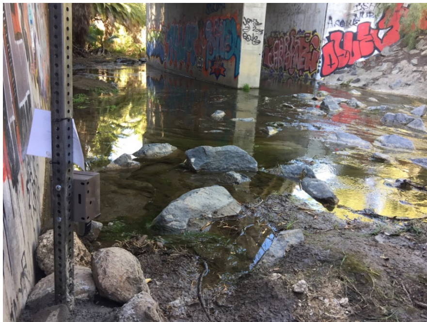
Photograph 8: View north from Camera 6 (located on the east side underneath Bridge 2) that shows both spans of Bridge 2. Brea Creek is relatively shallow here and large rocks have been cemented to the creek bottom for stability.
