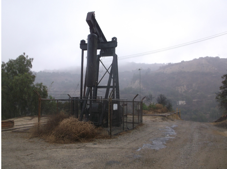
Plate 22: Brea Well #71, View East.
