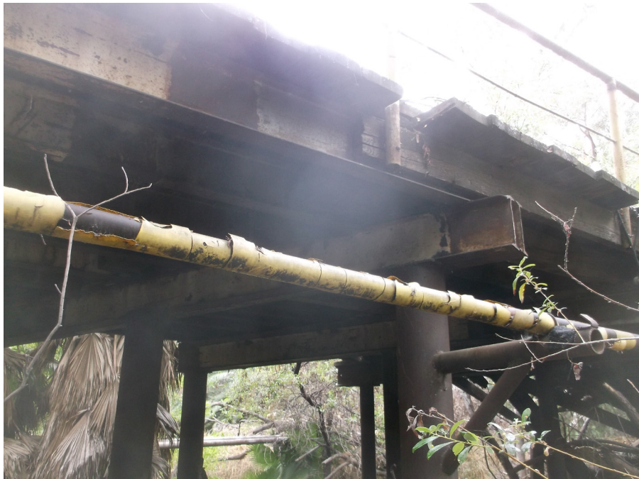
Plate 11: Abandoned Bridge from Below, View Southwest.
