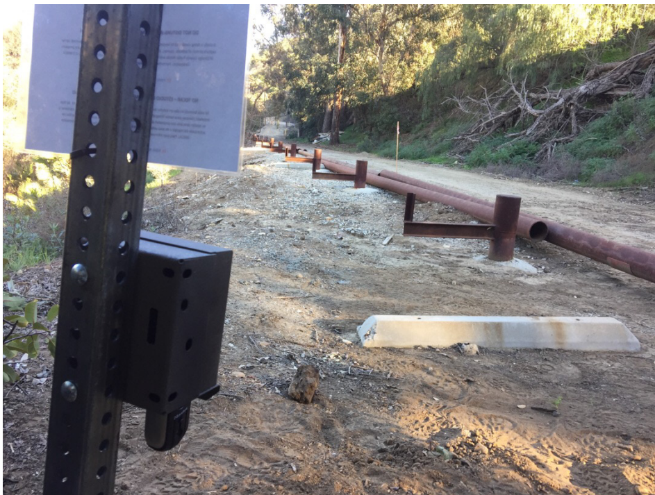
Photograph 10: View south across dirt road from Camera 8 (located at grade on the south side of Brea Boulevard) on the west side of Brea Creek and Bridge 3.
