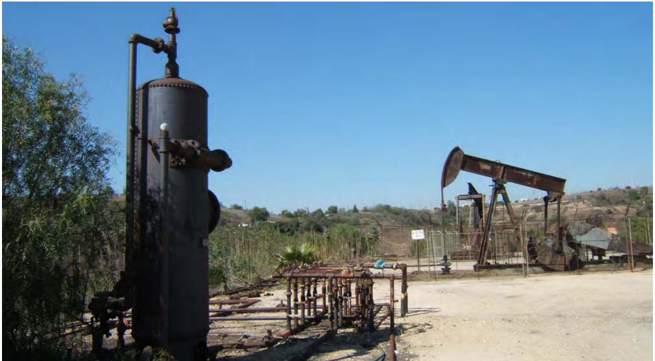
P5b3. Brea-Olinda Oilfield, facing N, 22 February 2006. Derricks, surge tank, and piping carry 1930s builders' plates.
