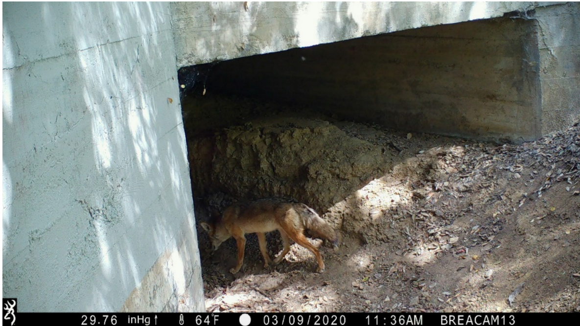
Photograph 9: Coyote walking into Culvert 3 from the south side of Brea Boulevard on Camera 13.
