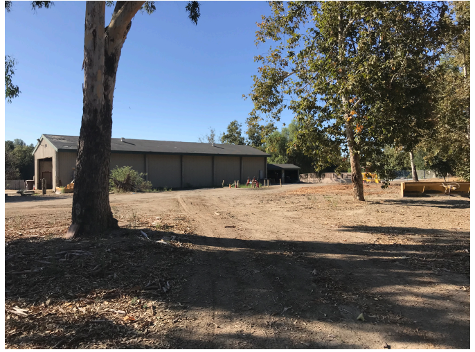
Existing barn located on the central-eastern portion of the property.
