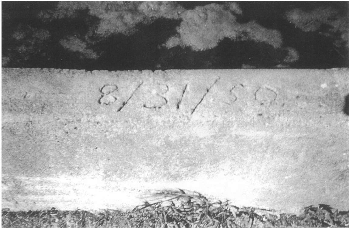
Figure 6. 1950s Water Trough (above) with Installation Date.
