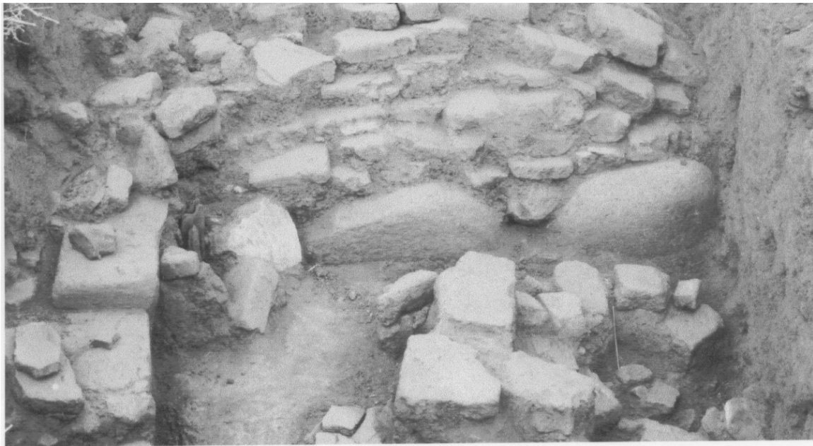
Figure 11. Unit 5, Ladrillo Courses.
