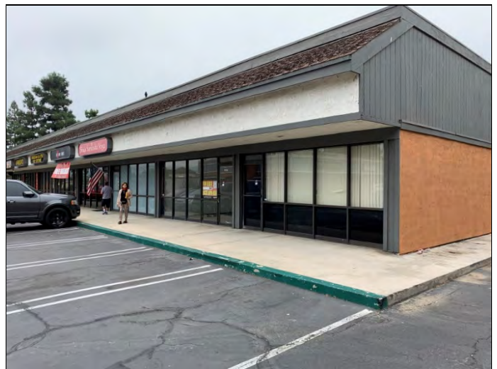
12. East side of the 19801-19819 Building, view facing southwest.
