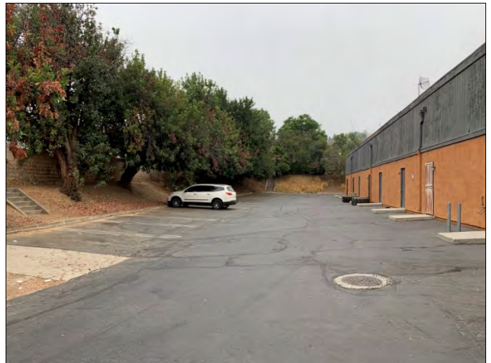
16. West side of the 19801-19819 Building, view facing north.
