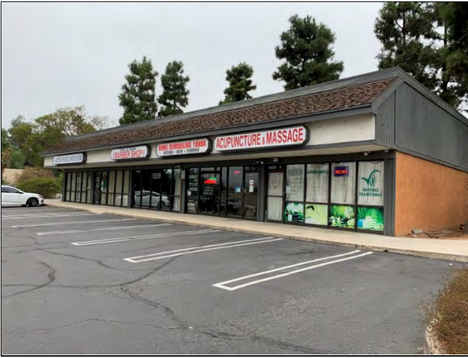
31. 19751-19761 Building, view facing northwest.
