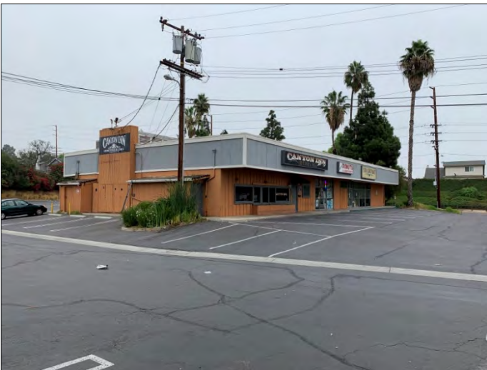
5. 6821-6829 Building, view facing northeast.
