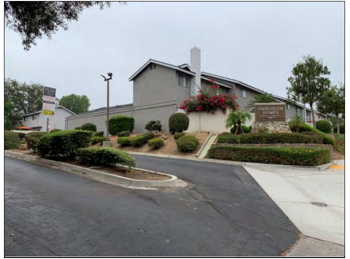
38. Adjacent properties to the north, view facing northwest.
