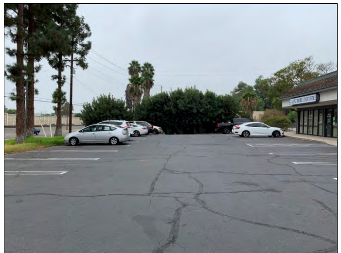
30. South side of the 19751-19761 Building, view facing west.
