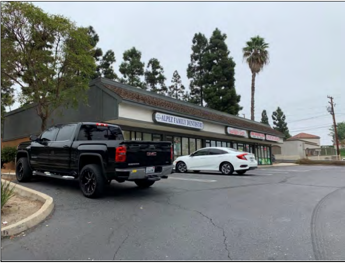
25. 19751-19761 Building, view facing northeast.
