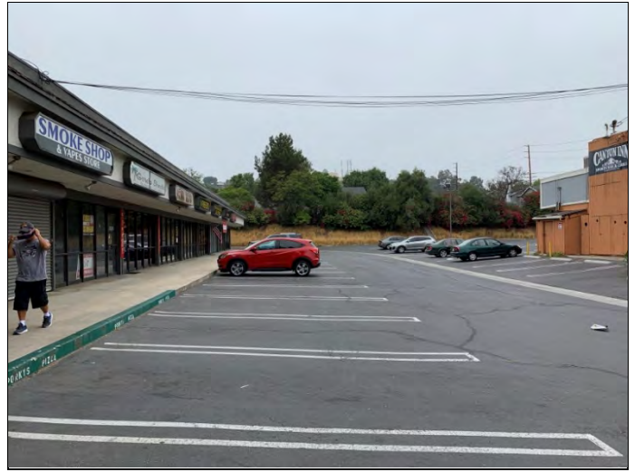
8. East side of the 19801-19819 Building, view facing north.
