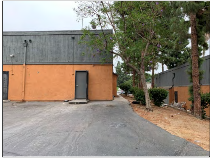
20. East side of the 19801-19819 Building, view facing east.
