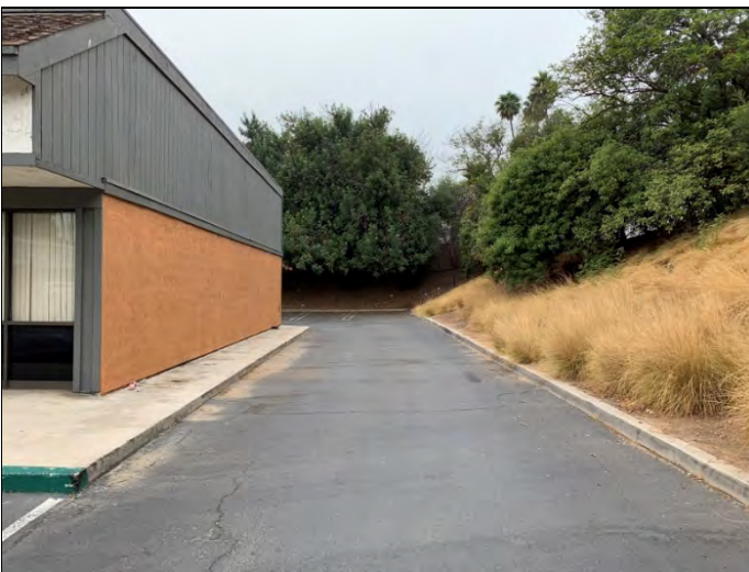
11. North side of the 19801-19819 Building, view facing west.
