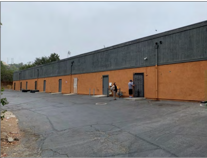
21. East side of the 19801-19819 Building, view facing northeast.
