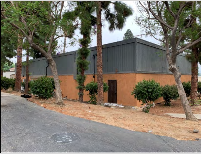
19. North side of the 19751-19761 Building, view facing southeast.
