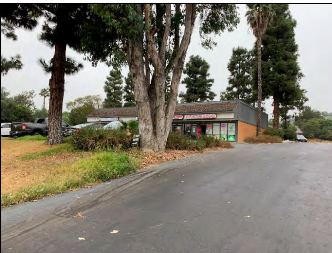
35. 19751-19761 Building, view facing northwest.
