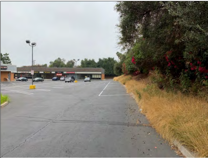
3. Subject property from the northeast corner of the site, view facing west.
