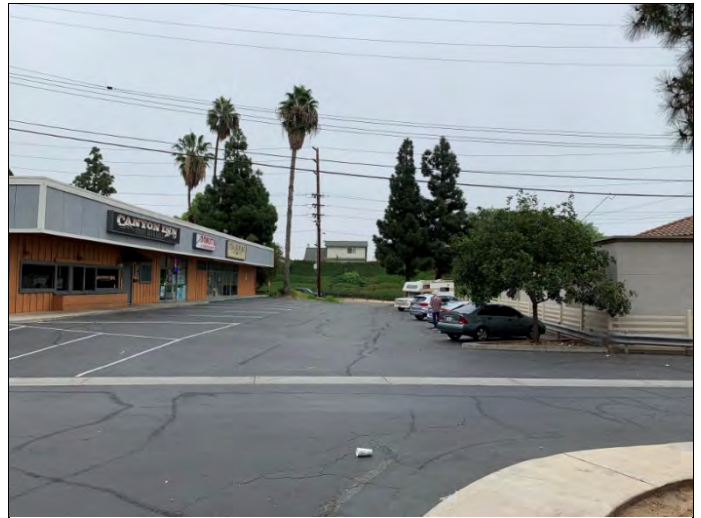
4. South side of the 6821-6829 Building, view facing east.
