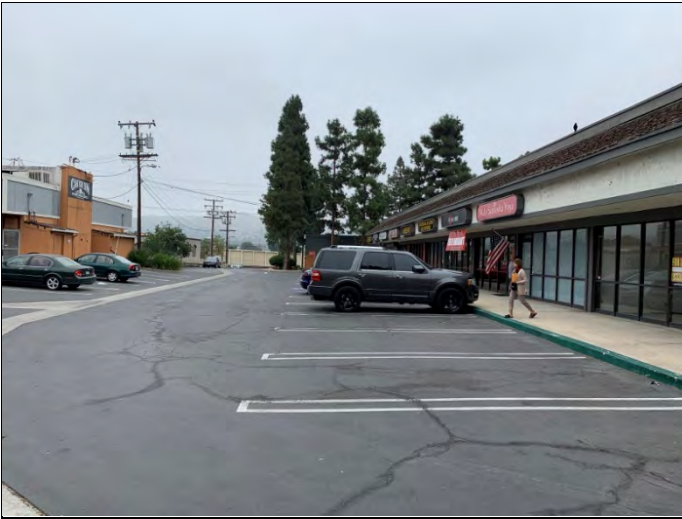
13. East side of the 19801-19819 Building, view facing south.
