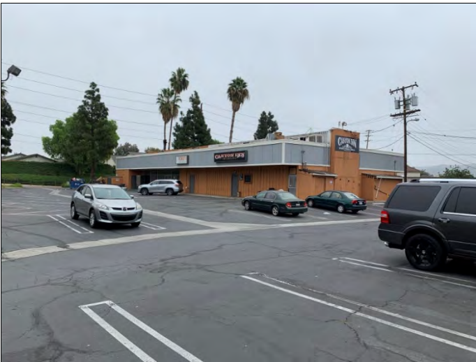
15. North side of the 6821-6829 Building, view facing southeast.
