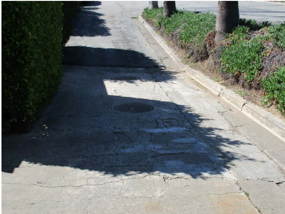
Photo 12 – Sewer manhole covers southwest of the clubhouse.
