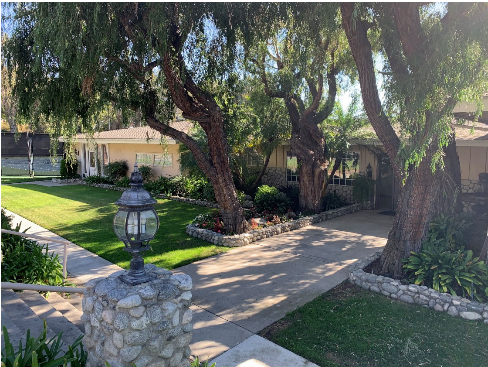
Figure 5-2 Clubhouse, northwest elevation, facing north
