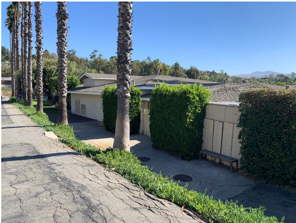
Figure 5-4 Clubhouse, northwest elevation, facing south
