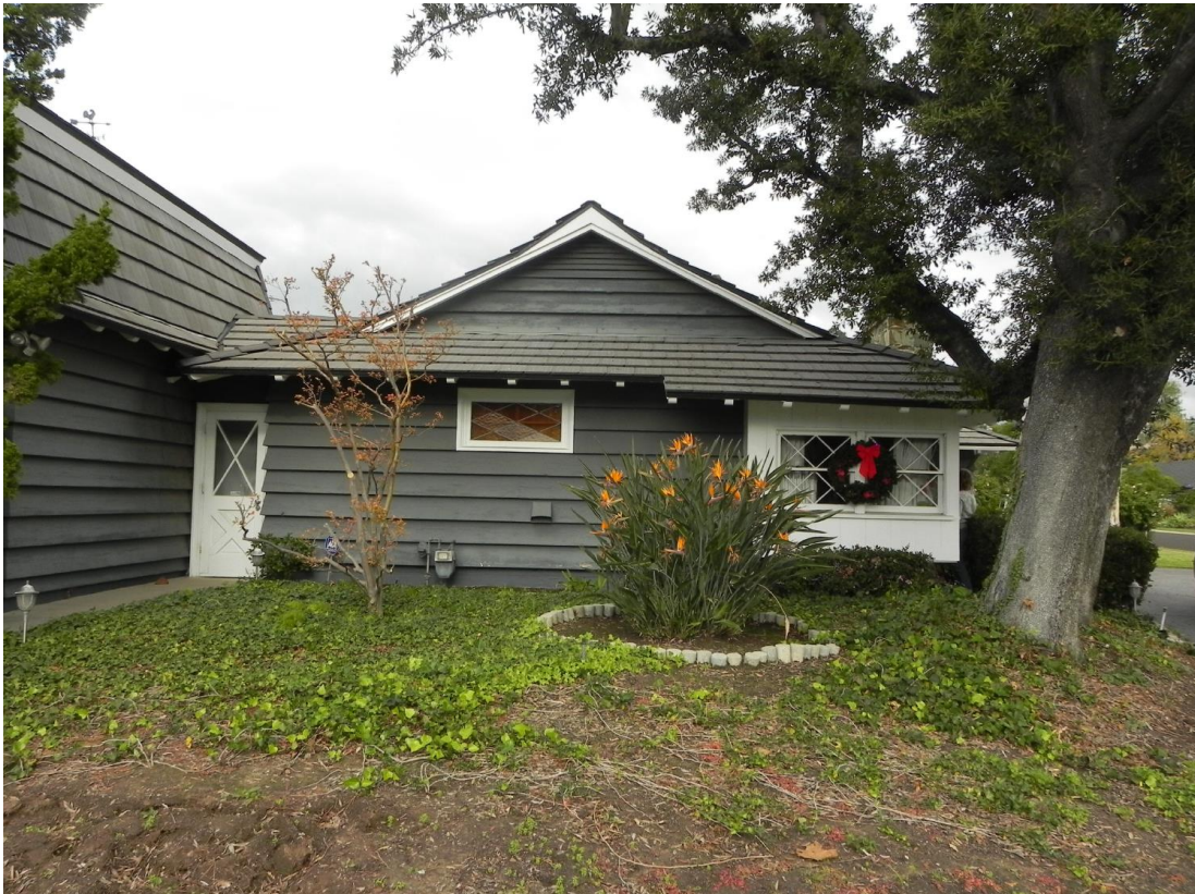
Facing north, toward affected area of residence. Breezeway on opposite side of white door.
