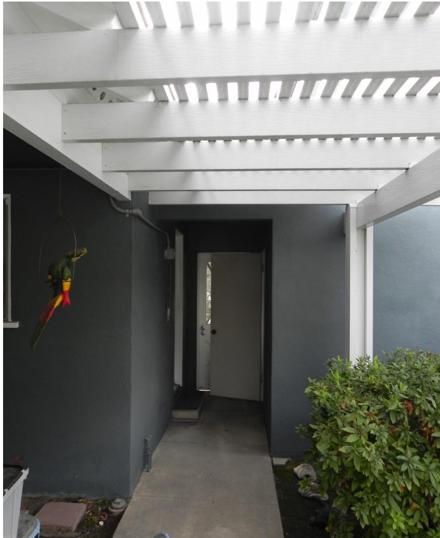
From interior of property, facing toward breezeway.
