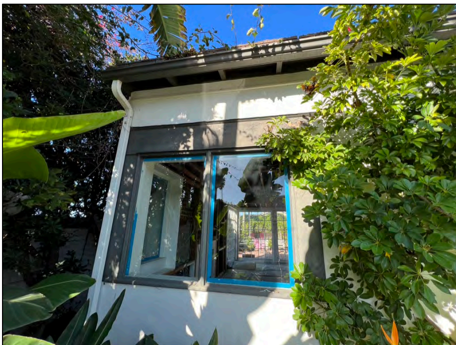
Photo 4. Southwest corner replacement windows and visible eave overhang.
