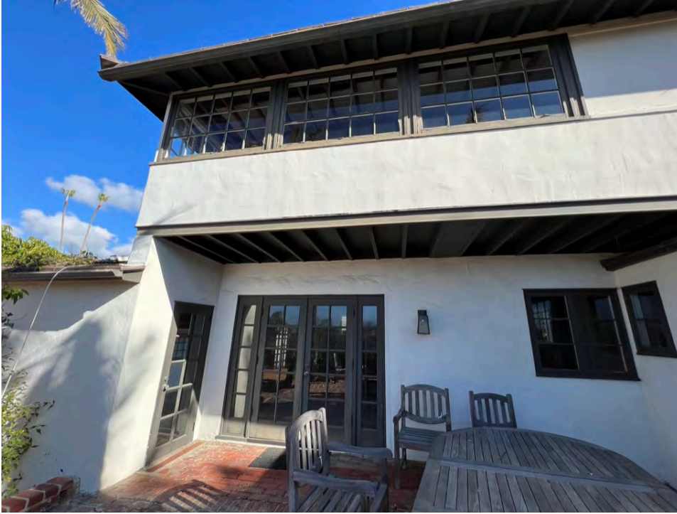
Photo 21. Main dwelling, west elevation fenestration at west-facing facades with non-original French doors, and inelegant placement of wood windows at the west-and-north-facing wall junction (at right).
