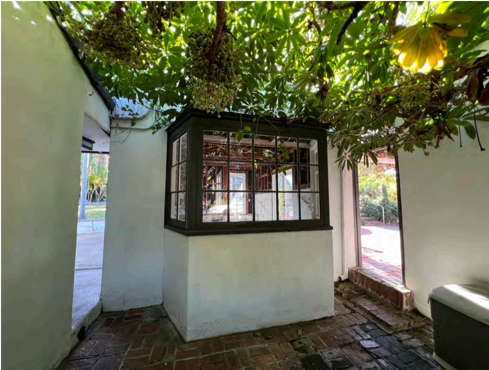
Photo 10. Main dwelling, north elevation of north addition.
