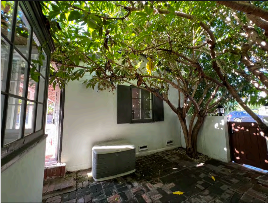
Photo 11. Accessory dwelling, east elevation and brick courtyard wall.
