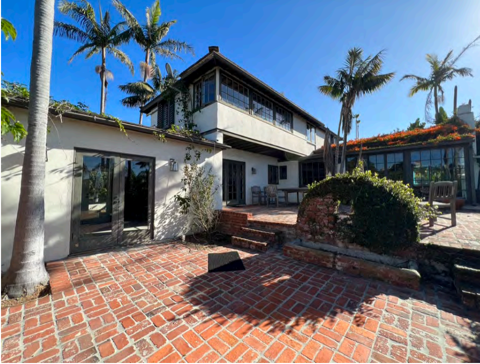
Photo 19. Main dwelling, west elevation, north-facing facade (at right) and west facing facade (at left), with north addition at far left. The enclosed 2nd level porch / balcony is demarcated by the windows.
