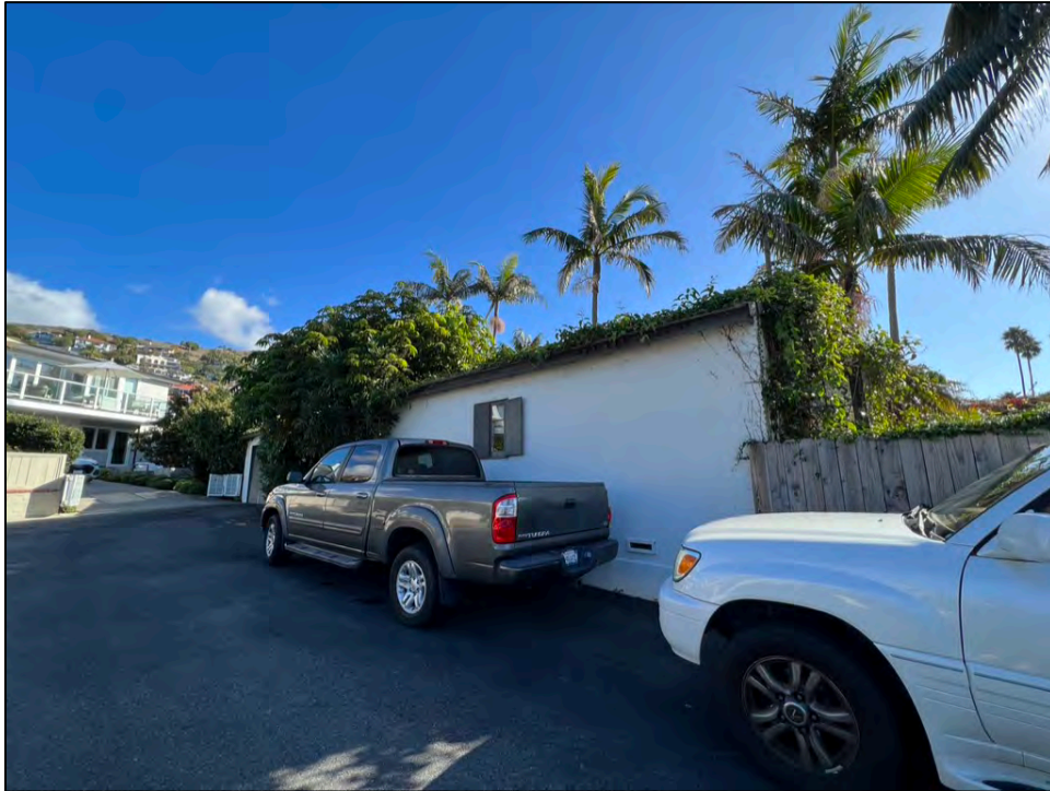
Photo 31. North lot line with accessory dwelling north elevation abutting the lot line.
