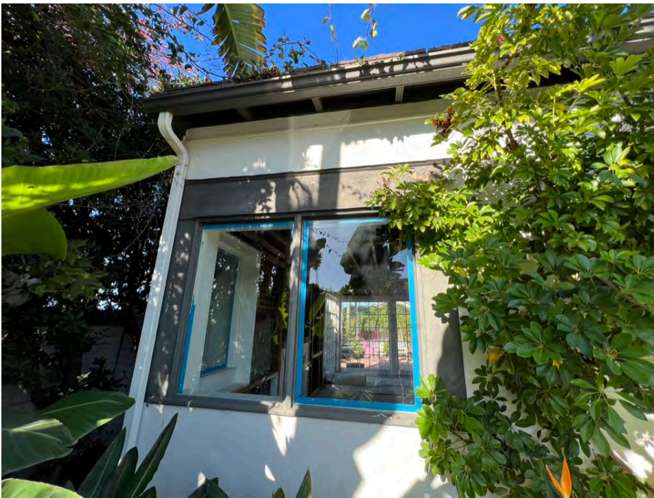
Photo 4. Southwest corner replacement windows and visible eave overhang.
