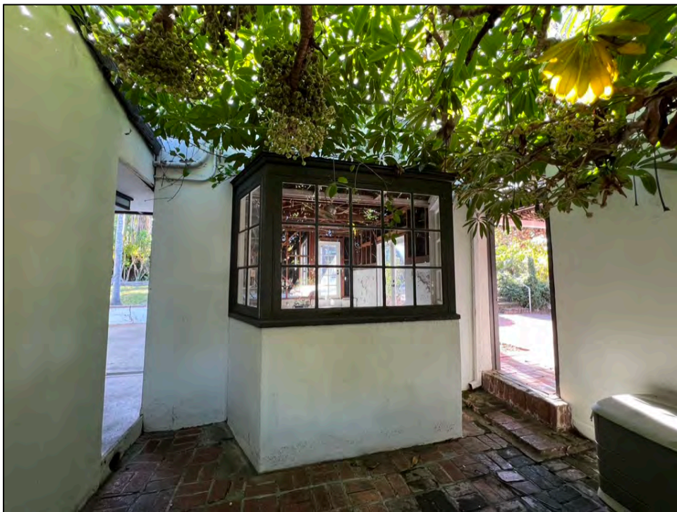
Photo 10. Main dwelling, north elevation of north addition.
