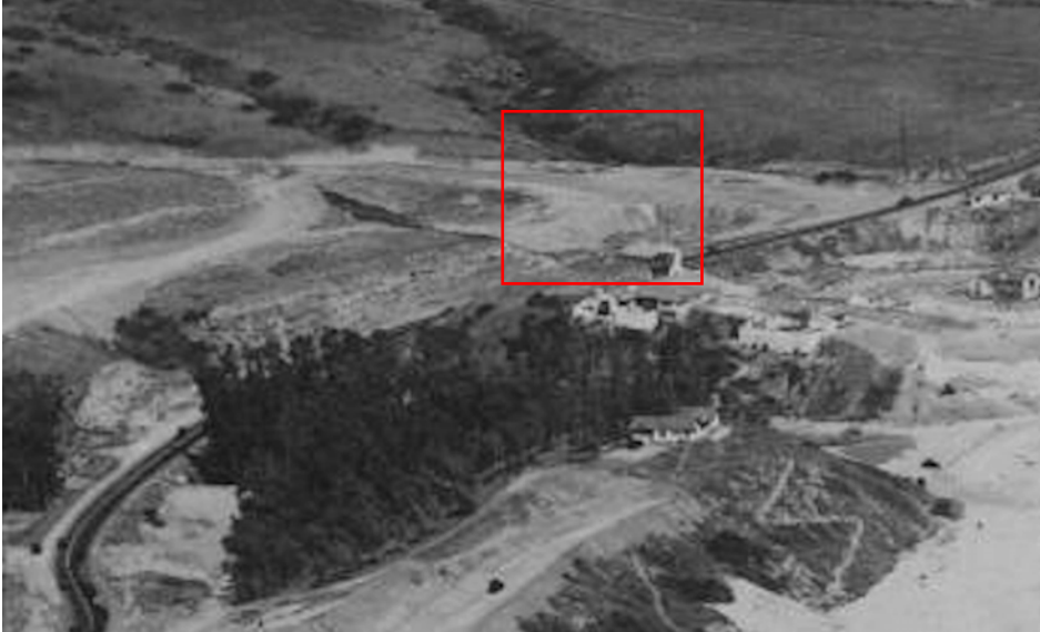
Figure 4. Detail view, 1931. Source: OC Public Libraries, Spence Air Photos via Calisphere. The 211 Emerald Bay property is vacant / undeveloped.
