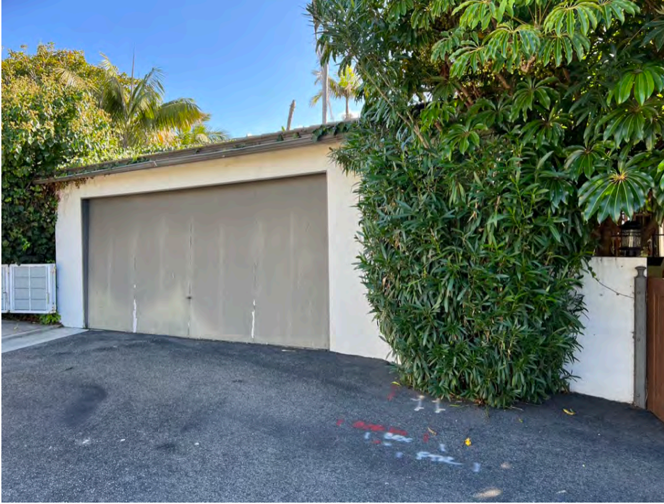
Photo 33. North lot line, north elevation of detached garage, sited east of the courtyard gate.
