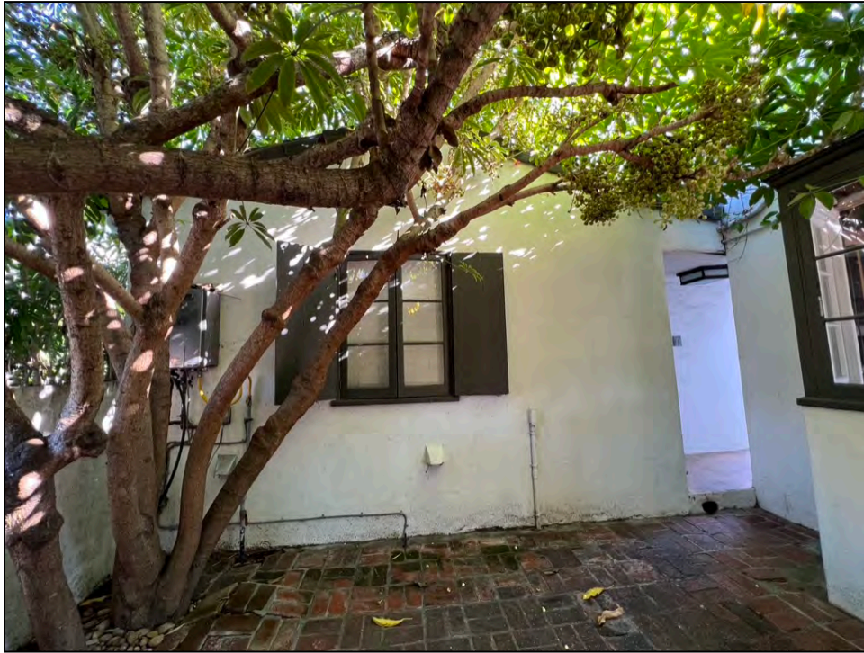
Photo 9. Detached garage, west elevation.
