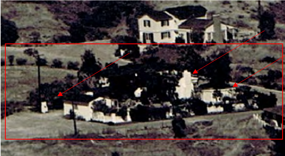
Figure 13. Detail view, ca. 1940-1945. Source: Laguna Beach Historical Society. The 211 Emerald Bay property is developed in this view but was later altered. Subsequent to this photo, an ancillary building or structure west of the home was removed, the existing detached garage was constructed, and the chimney at the west elevation of the main dwelling appears to have been altered as the chimney appears larger than that depicted today, or the white walls may show the original northwest corner of the home, prior to the glass wall enclosure.
