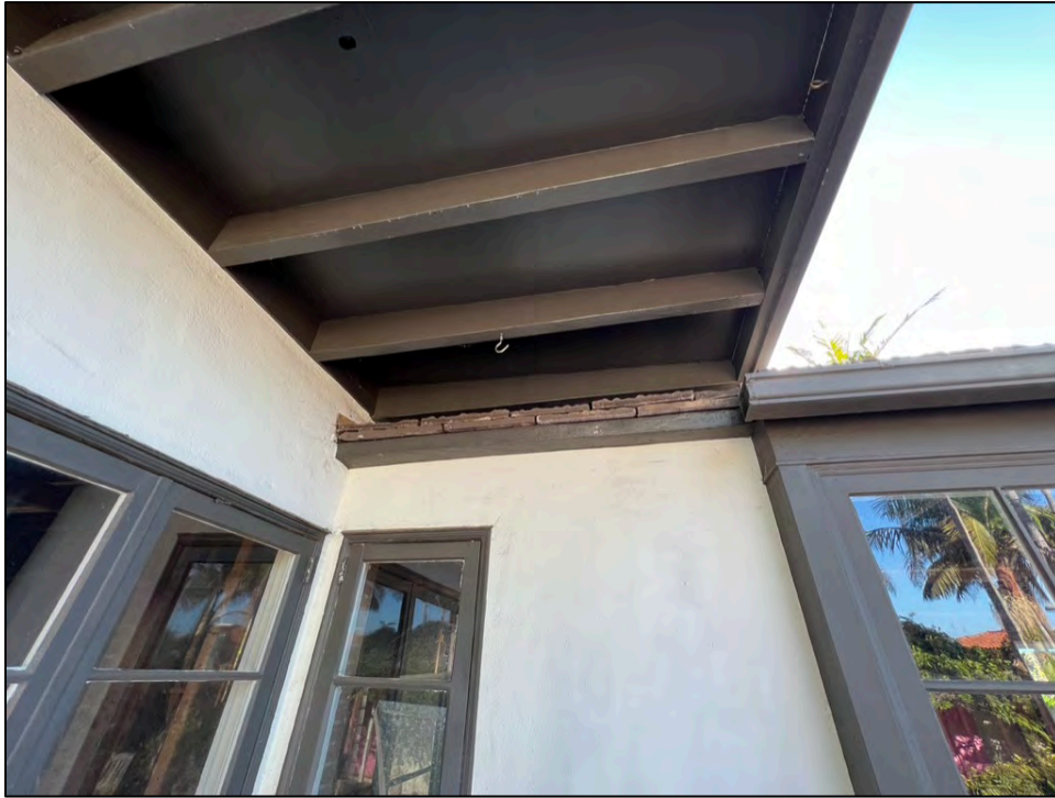
Photo 23. Main dwelling, west elevation, west-and-north-facing wall junction.
