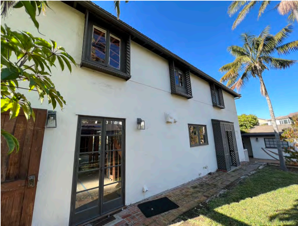
Photo 6. Main dwelling, east elevation.
