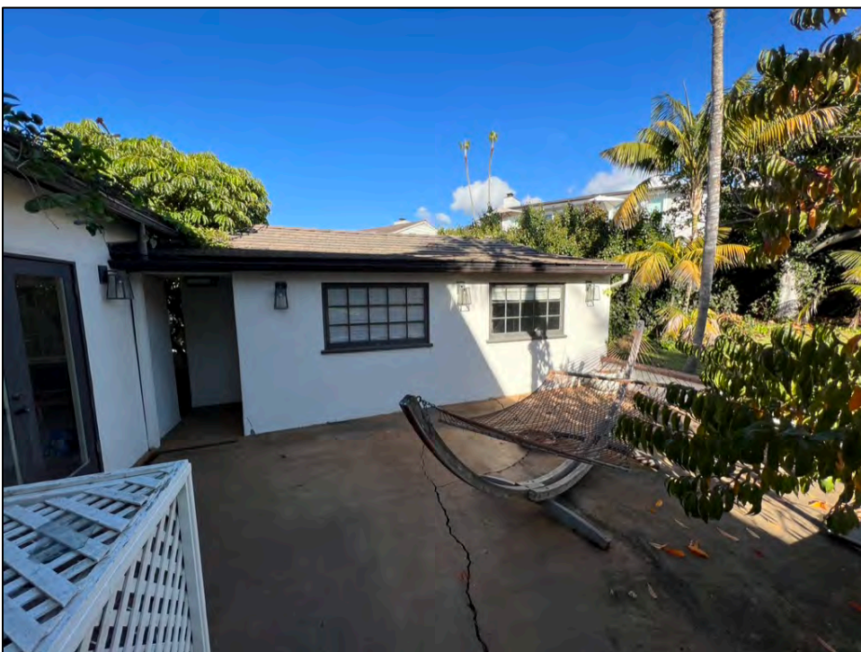
Photo 8. Detached garage, south elevation.
