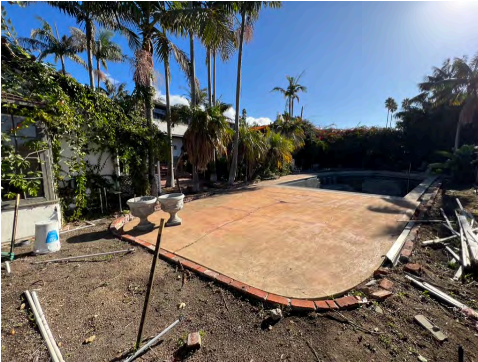
Photo 16. Hardscape and Landscape view, northwest corner (Lot 6).
