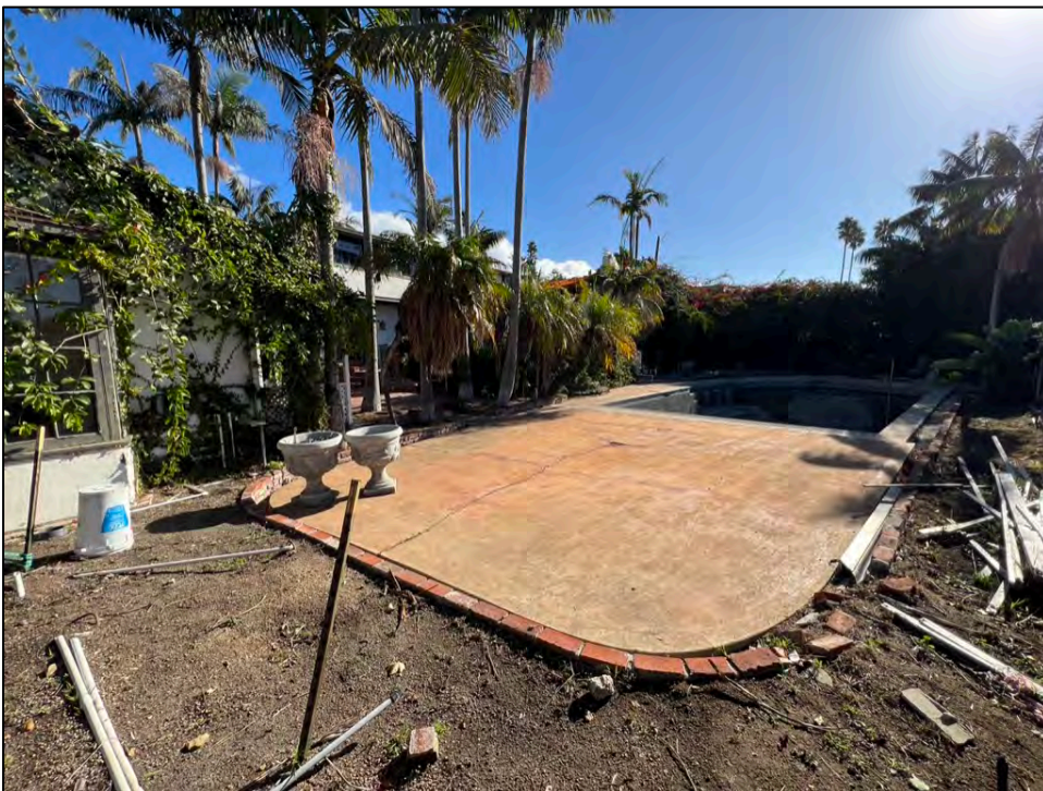
Photo 16. Hardscape and Landscape view, northwest corner (Lot 6).
