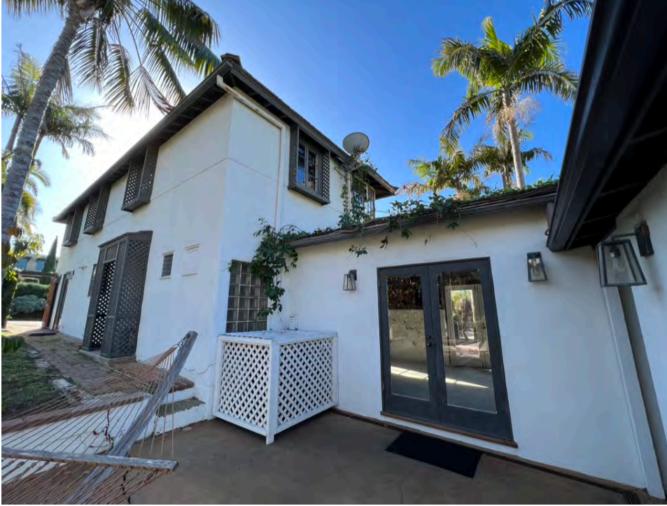
Photo 7. Main dwelling, east elevation with the north elevation addition.
