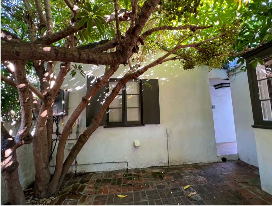
Photo 9. Detached garage, west elevation.
