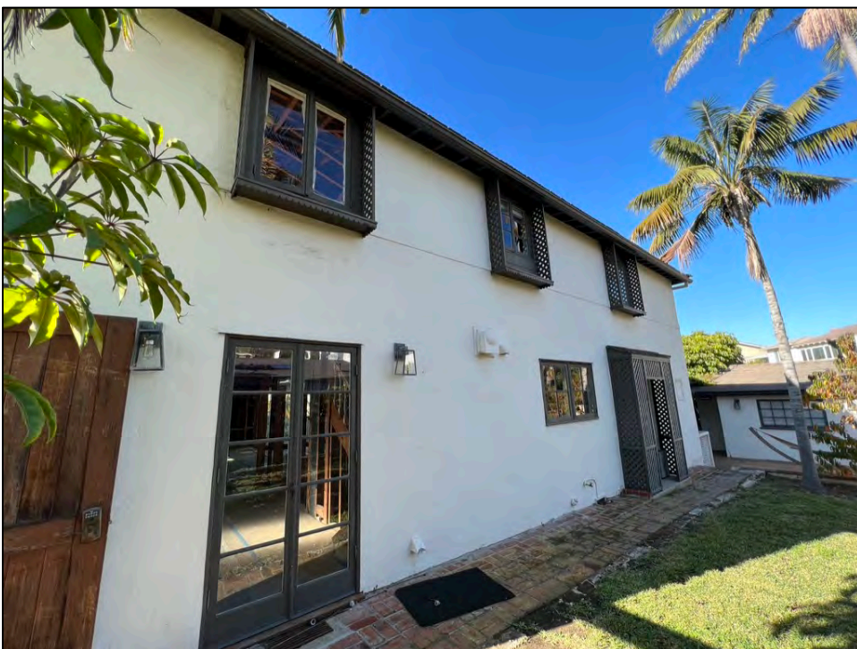
Photo 6. Main dwelling, east elevation.
