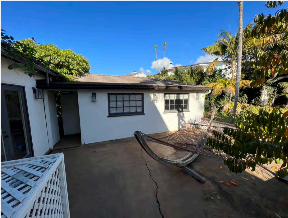
Photo 8. Detached garage, south elevation.
