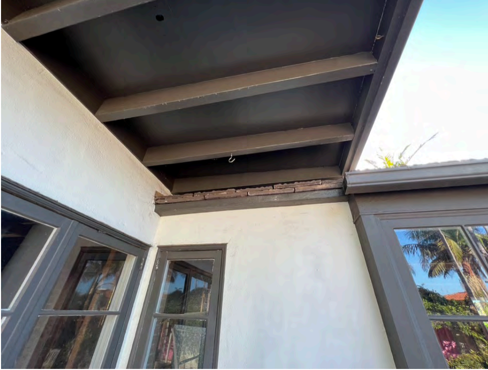
Photo 23. Main dwelling, west elevation, west-and-north-facing wall junction.
