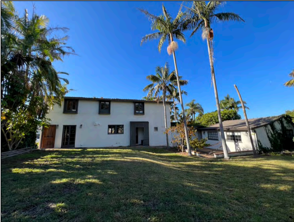
Photo 5. Main dwelling, east elevation with north elevation addition and detached garage addition.
