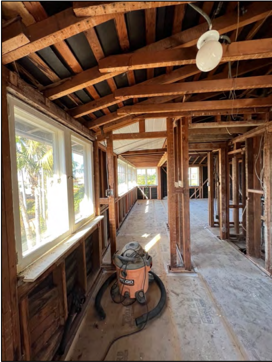
Photo 27. Main dwelling, interior view of original 2nd level porch / balcony enclosed.
