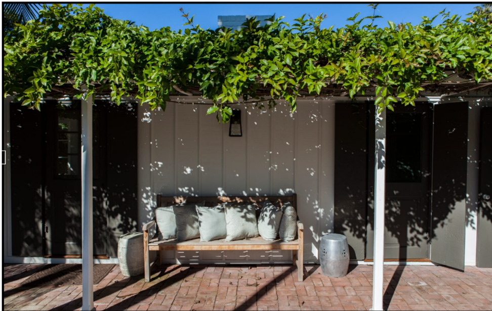
Figure 8. The board-and-batten siding and wooden posts supporting the pergola at the rear of the main house, view looking north. Source: Compass real estate listing, 2018.
