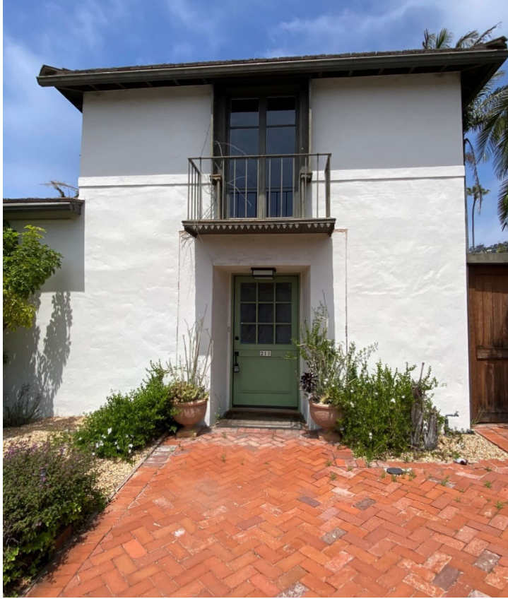
Figure 4. Primary entrance with an original Dutch-door. South elevation, view looking north. Source: ESA 2023.
