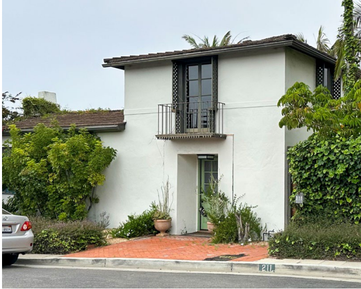
Photo 3- View of the stucco chimney on the northwest elevation and Juliette balcony with wrought-iron railing and decorative scalloped detailing on the southeast elevation. The French doors above the main entrance are a pair of original 4-lite, full-height wood casement windows with original wood lattice frames. Other windows on the second story include original wood-frame multi-lite casement windows, also with original wood lattice frames as seen on this photo on the northeast elevation. Source: ESA 2023.
