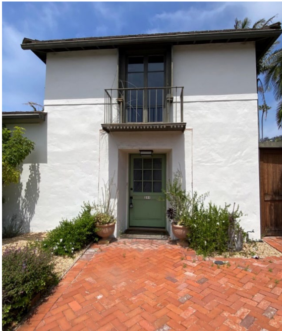
Photo 6- Primary entrance with an original Dutch-door. Southeast elevation, view looking northwest. Source: ESA 2023.
