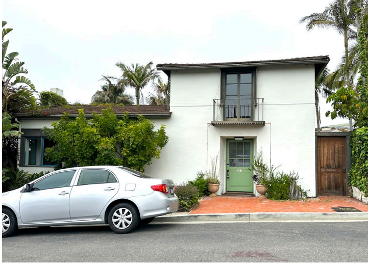
Photo 1- A Mediterranean Revival style residence at 211 Emerald Bay. The facade's two-story volume is vertically centered with a ground floor entrance surmounted by a Juliette balcony with original details. Southeast elevation, view looking northwest. Source: ESA 2023.
