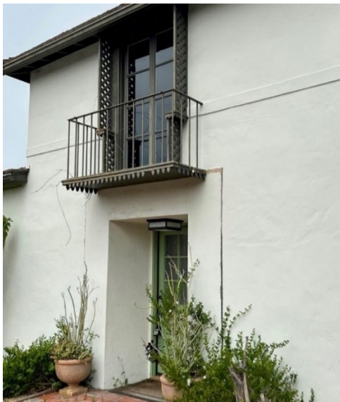
Photo 4- Detail of the stucco exterior, belt course, and Juliette balcony with original wrought-iron railing and decorative scalloped detailing above the entrance. Southeast elevation, view looking north. Source: ESA 2023.
