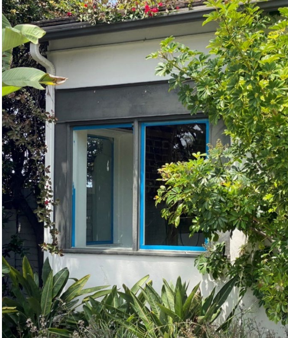
Photo 7- Detail original window opening with replacement window on the southeast elevation, view looking north. Source: ESA 2023.
