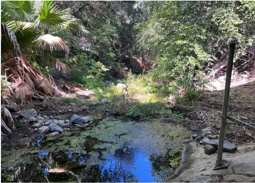
Photograph 3: View looking west at Santiago Creek underneath Modjeska Grade Road Bridge. Latitude 33.708747°, Longitude -117.636344°.
