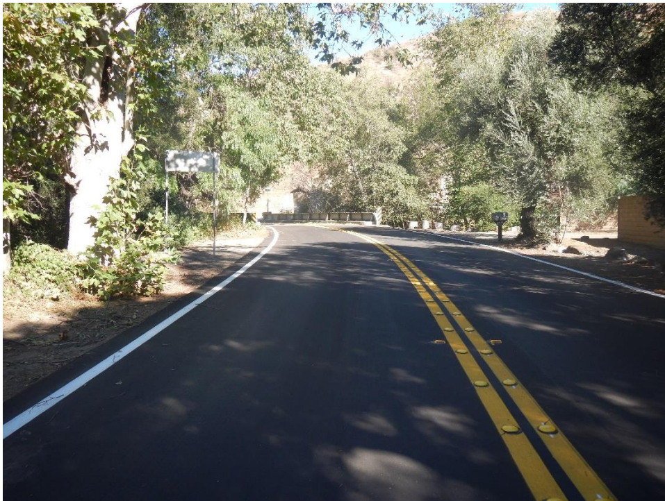
Photograph 8: Looking north along Modjeska Grade Road at the northern end of the project site.
