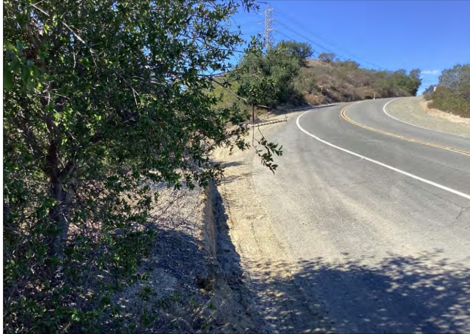
Photograph 1. Overview of the southern end of Modjeska Grade Road. View to northwest, October 2022
