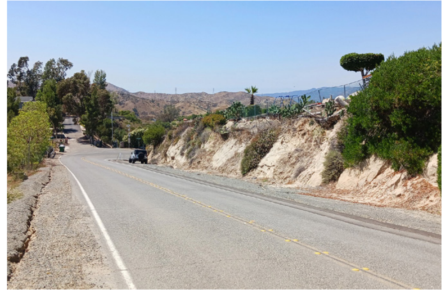
Looking northwest along the southbound shoulder of Modjeska Grade Road, approximately 300 feet south of the Canyon Heights Drive and Modjeska Grade Road intersection.
