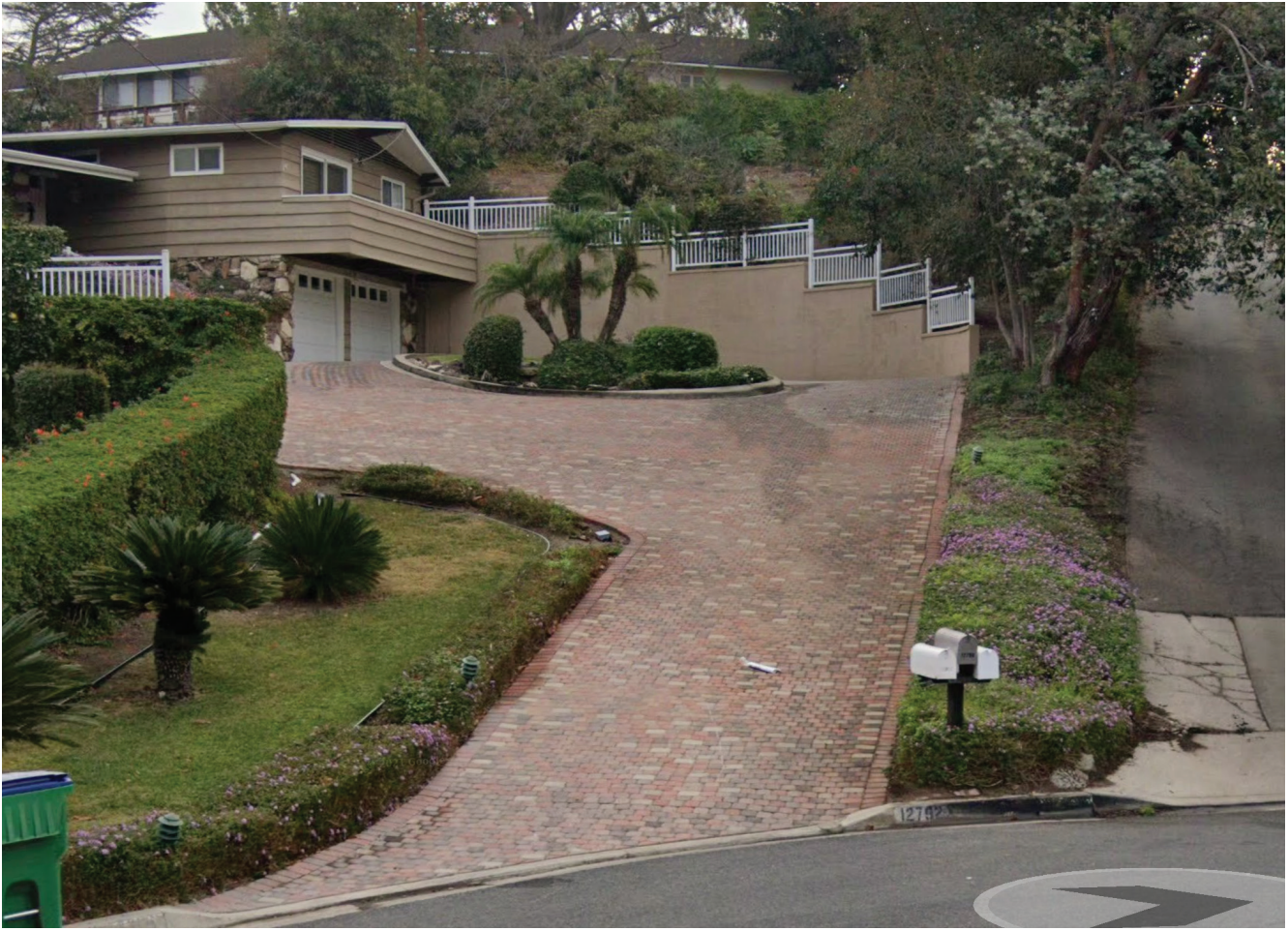
12899 Bonita Heights Dr, North Tustin over 10' wall plus barrier atop
