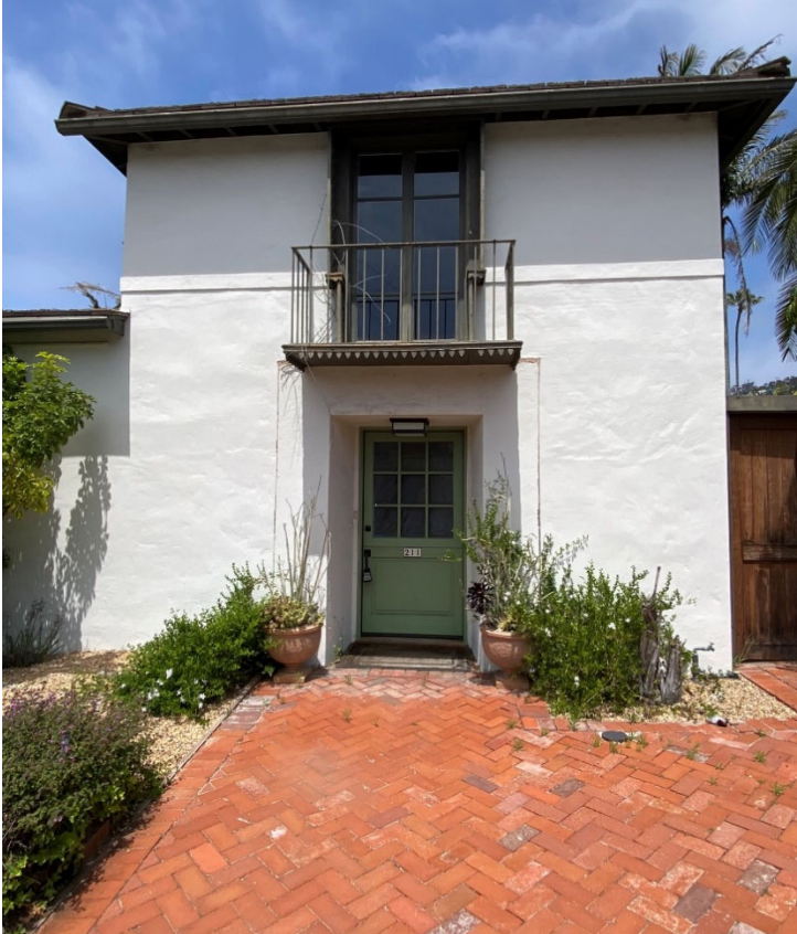
Figure 4. Primary entrance with an original Dutch-door. South elevation, view looking north. Source: ESA 2023.
