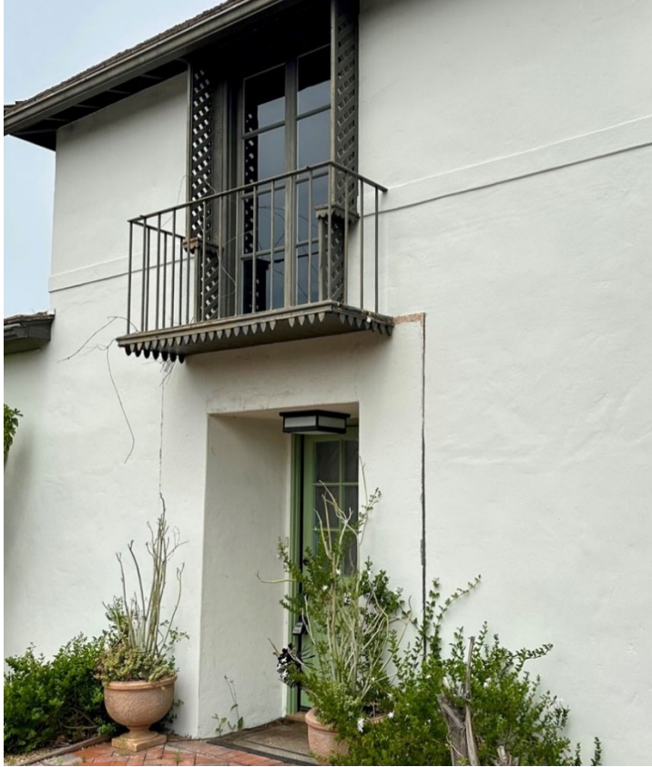
Figure 2. Detail of the stucco and original wood ornamental design around the entrance. The wooden lattice under the balconette that surrounded the entrance has been removed. South elevation, view looking northwest. Source: ESA 2023.
