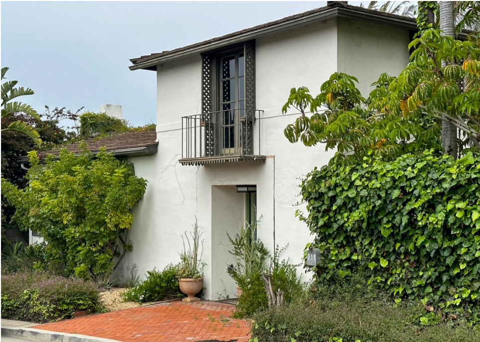
Figure 1. 211 Emerald Bay south elevation, view looking northwest. Source: ESA 2023.
