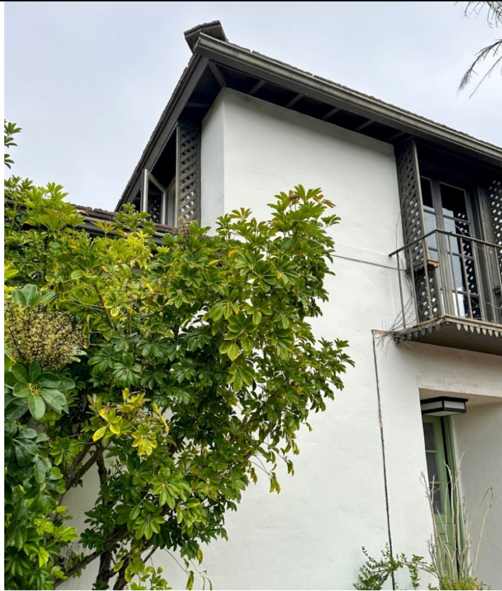
Figure 3. Details of overhanging roof eaves and wood lattice around the windows. South elevation, view looking northeast. Source: ESA 2023.
