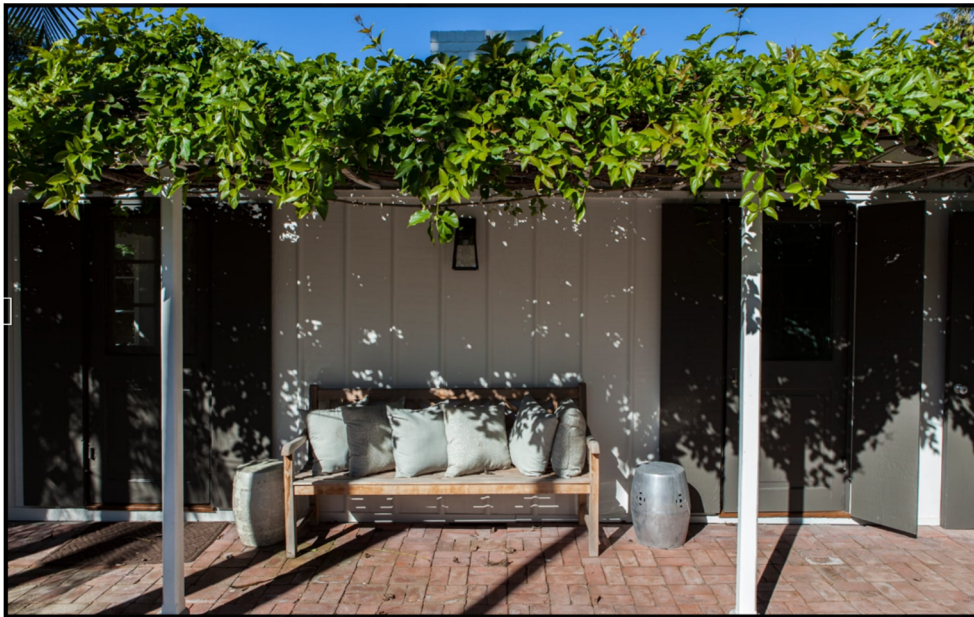
Figure 8. The board-and-batten siding and wooden posts supporting the pergola at the rear of the main house, view looking north. Source: Compass real estate listing, 2018.
