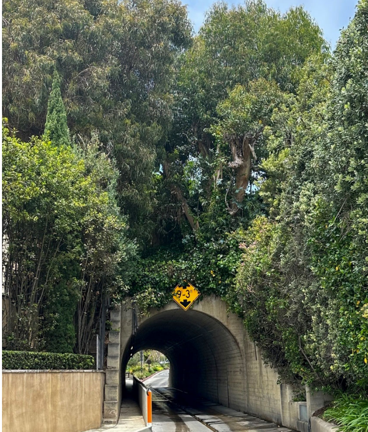
Figure 33. Historic tunnel connecting the Emerald Bay tracts on both sides of the Coast Highway, with landscaping above. Source: ESA 2023.
