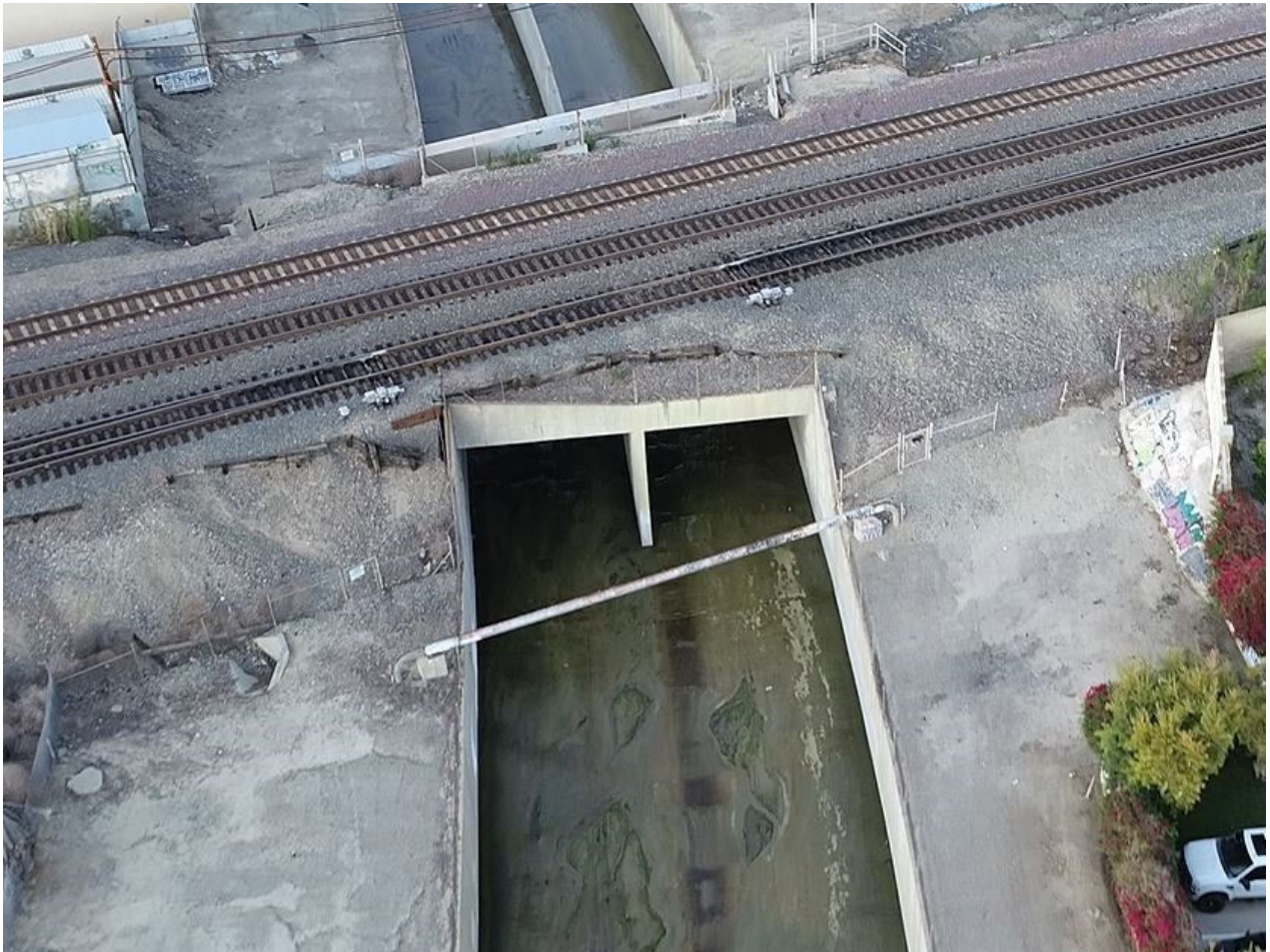
BNSF/Metrolink Corridor over Coyote Creek (looking upstream from downstream side)
