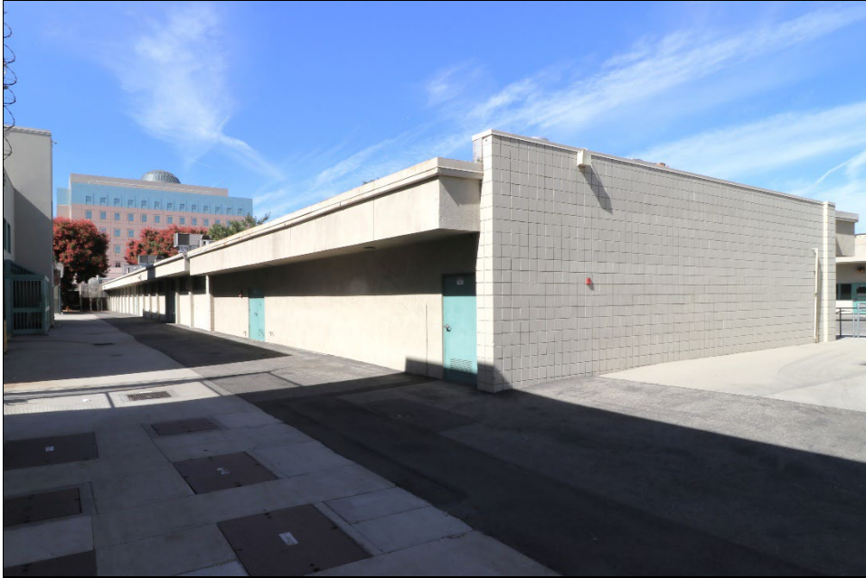
View northwest, 10/21/2024. Photo #9145.
