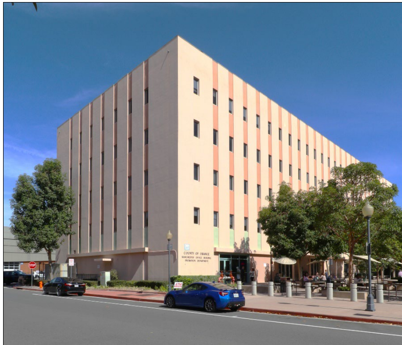
Building 27, view northeast (10/21/24)
