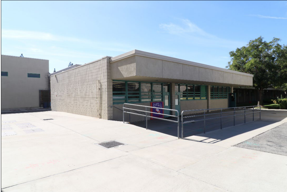
View southwest, 10/21/2024. Photo #9141.
