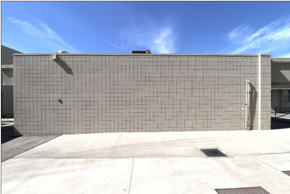
View west, 10/21/2024. Photo #9144.
