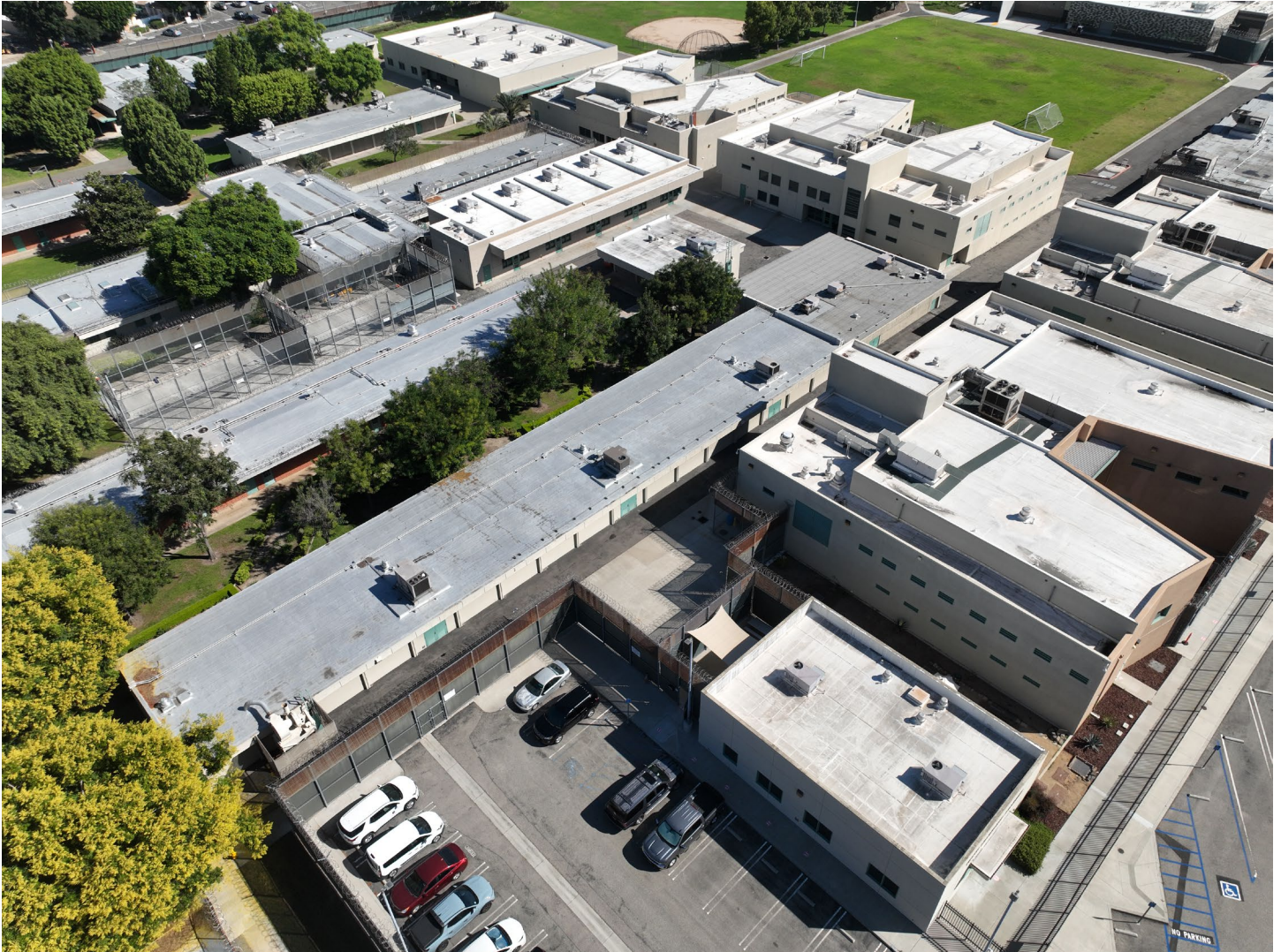
View northeast. At the top of the photo, left of center, is the library and office, Building #12. At the lower left is Building #11 (1968) and beneath that is the addition to Building #5, with SRA 2 and SRA 3 adjacent to it and Building #28. Refer to the Building Map on Continuation Sheet 23.
