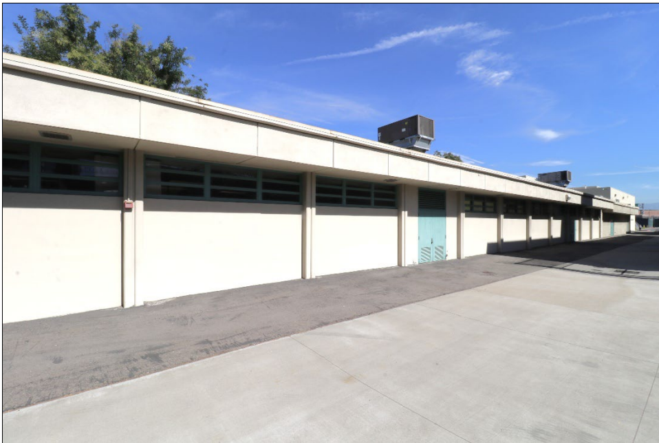
View northeast, 10/21/2024. Photo #9146. The addition is at the far right of the photo.
