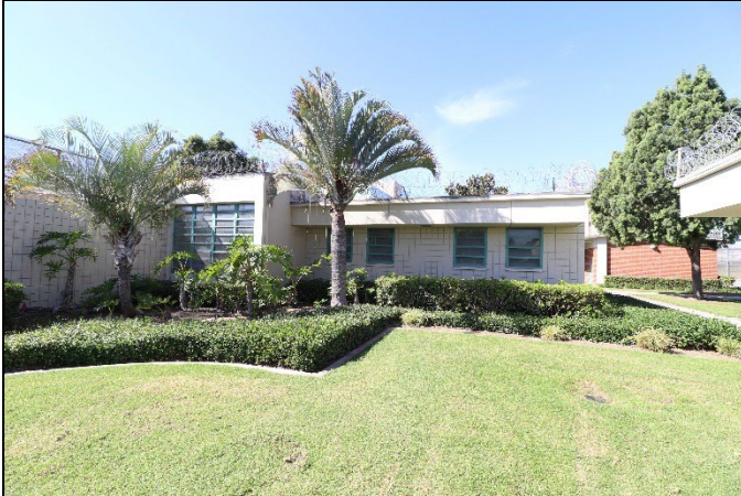
Building #5, Unit I, photo #9103, view west (10/21/24).
