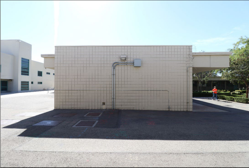
View S, 10/21/2024. Photo #9121. North elevation.
