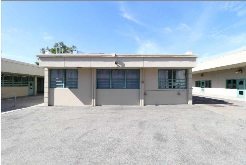
View W, 10/21/2024. Photo #9120. Rear of Building #14.
