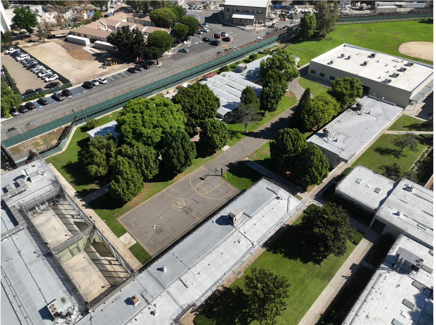
View east-northeast. All the buildings seen here are scheduled for Phase I demolition: two wings of Building #5, and Buildings #9, #10, #11, and #12. Refer to the Building Map on Continuation Sheet 23.
