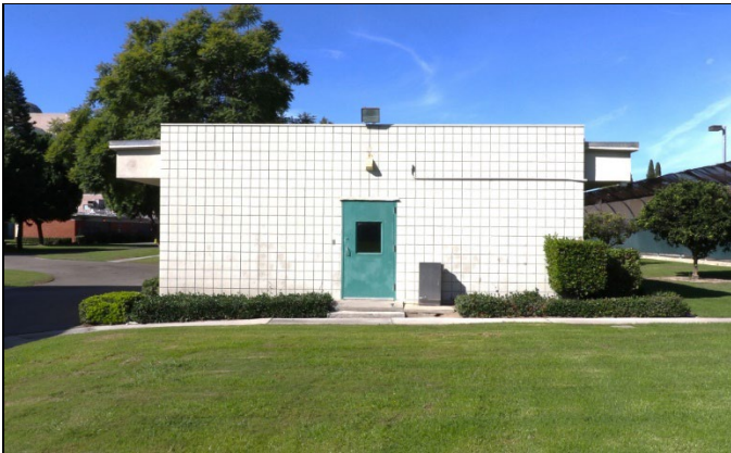
View West. 10/21/2024; Photo #9077. Building #9, Living Unit S (1968).
