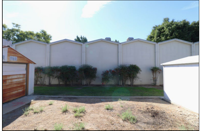
View south. 10/21/2024; Photo #9089. Building #9, Living Unit S (1968).
