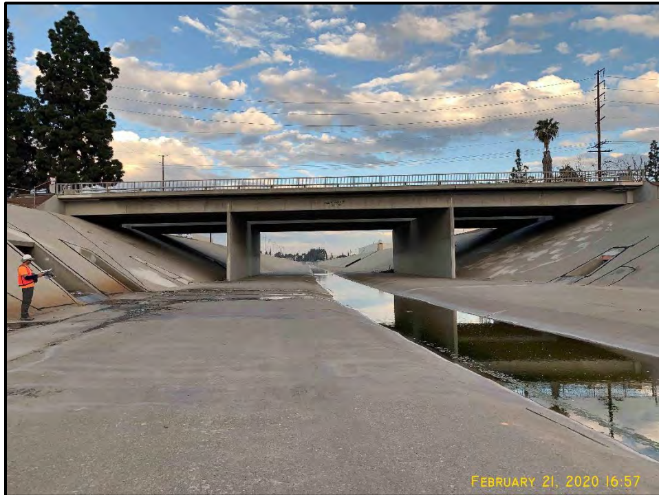
Photo 2. Segment O. Coyote Creek west of Valley View Boulevard. Water is present in the low-flow channel; in many areas of the channel the OHWM was determined by water staining (visible center left). View is upstream, looking east at the Valley View undercrossing.
