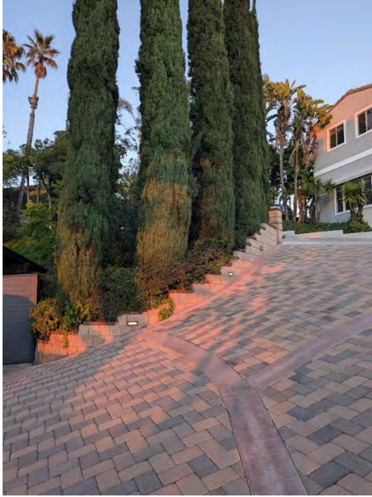
Bottom of Existing Driveway
