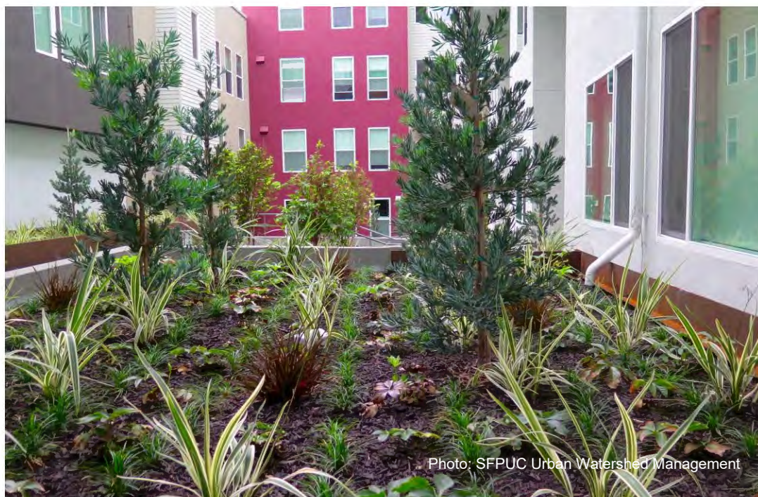
Figure 3. Downspout to mulched flow-through planter bed in project courtyard.
