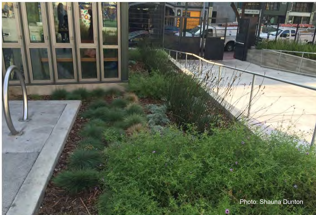
Figure 2. Mulched landscape area adjacent to permeable concrete at a public park in San Francisco.
