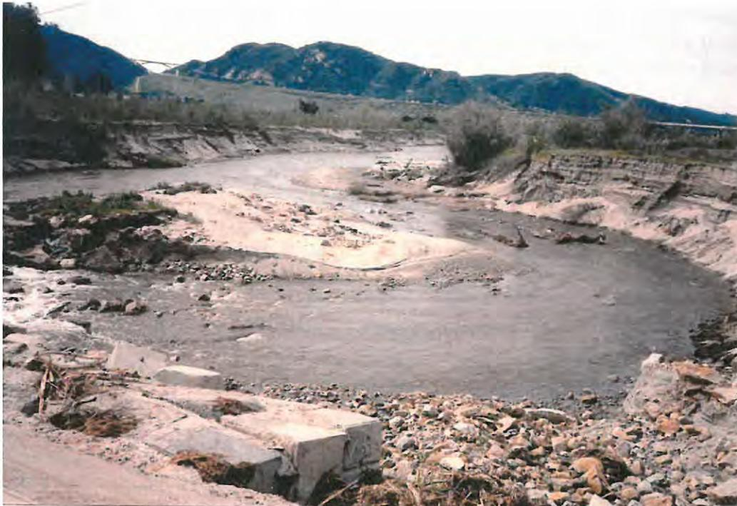
Figure 3. San Luis Rey River downstream of check dam at Shearer Crossing near Escondido, California. Channel responses to sediment deficit include degradation, development of more sinuous course, and coarsening of bed material
