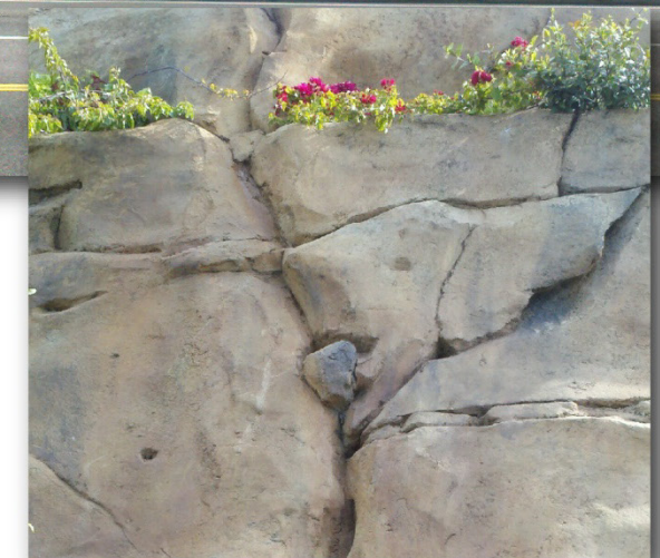
Shotcrete Retaining Wall
