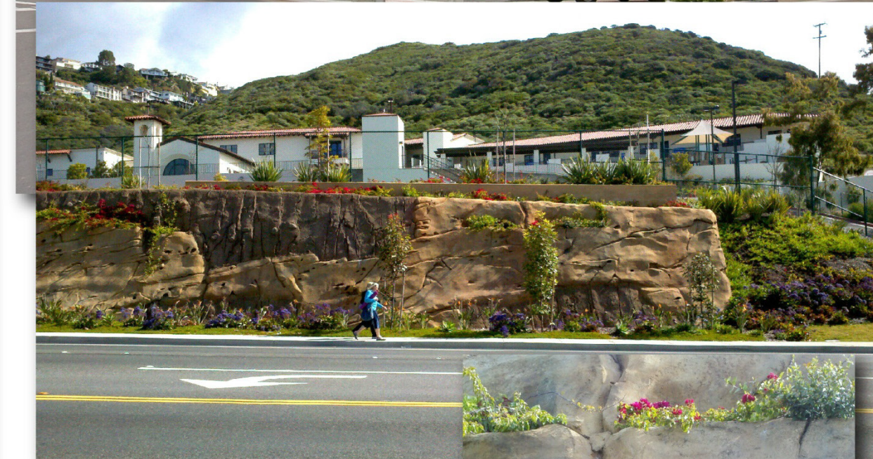
Shotcrete Retaining Wall
