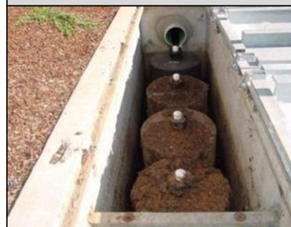
Cartridge Media Filter Source: Contech Stormwater Solution, Inc.
