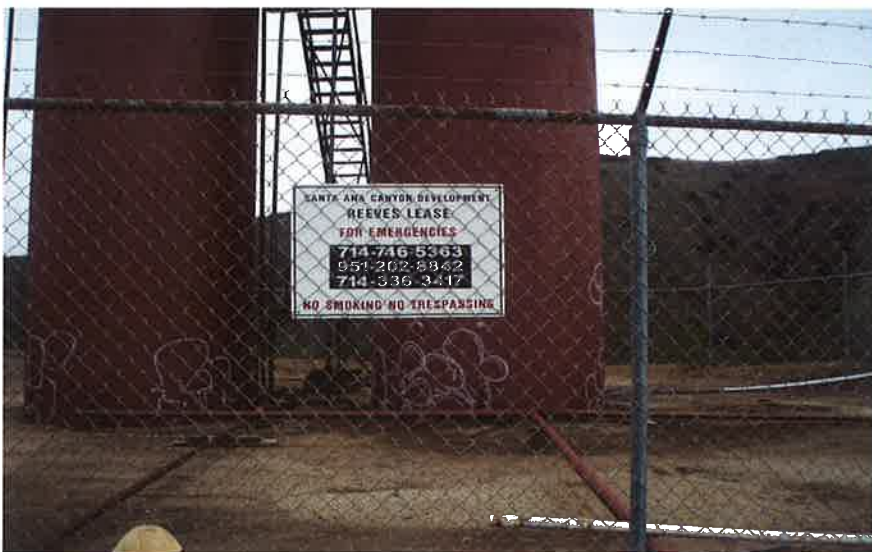
Tank Farm Adjacent To Reference Well Site #5
