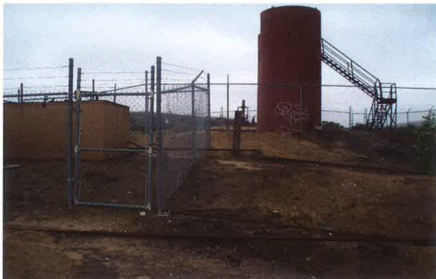
Tank Farm Adjacent To Reference Well Site #5
