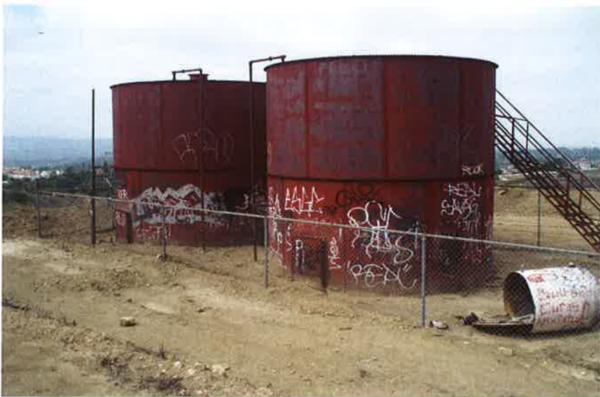
Tank Farm Adjacent To Reference Well Site #1
