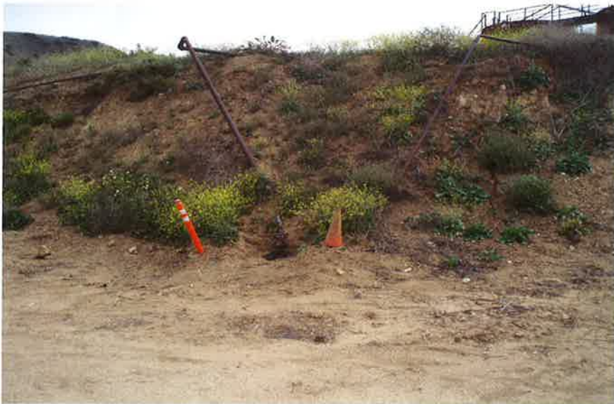
Tank Farm Adjacent To Reference Well Site #1
