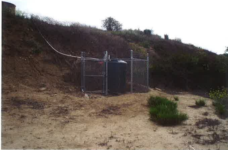
Tank Farm Adjacent To Reference Well Site #1
