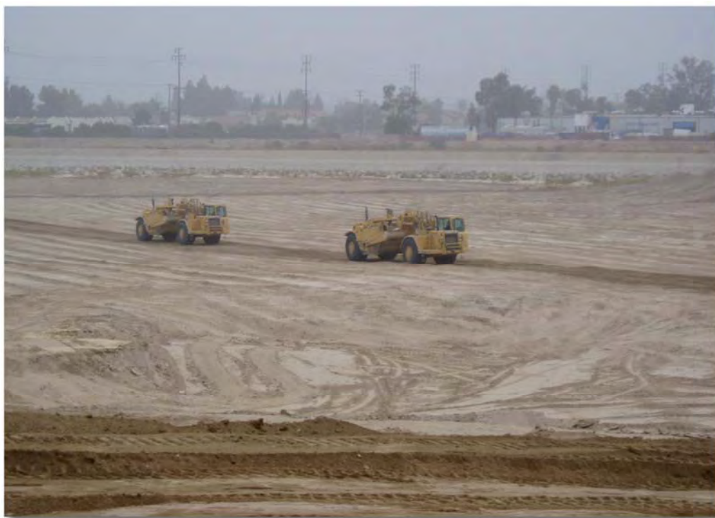
FIGURE 4-6 CLEANING OF RECHARGE BASINS
