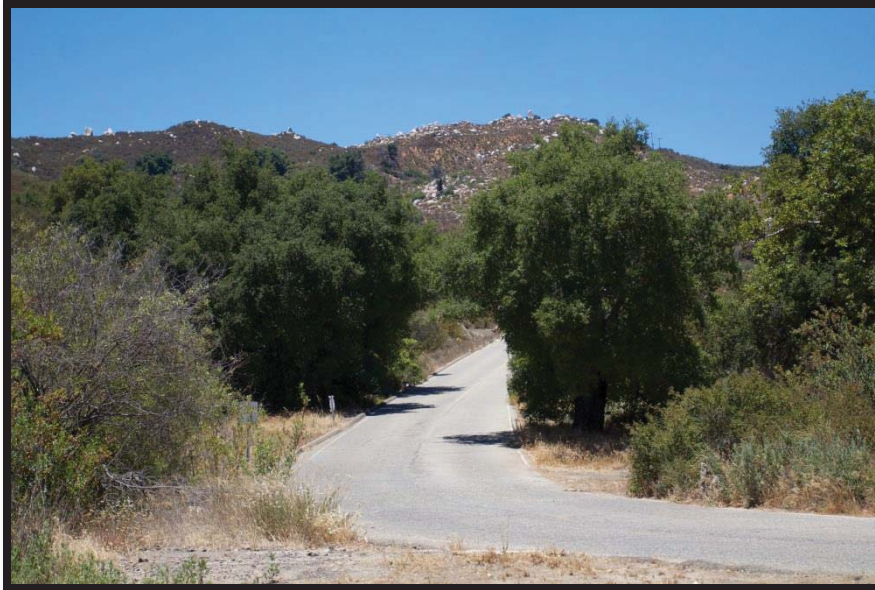
Photograph 3 – View of mature oaks along long canyon road
