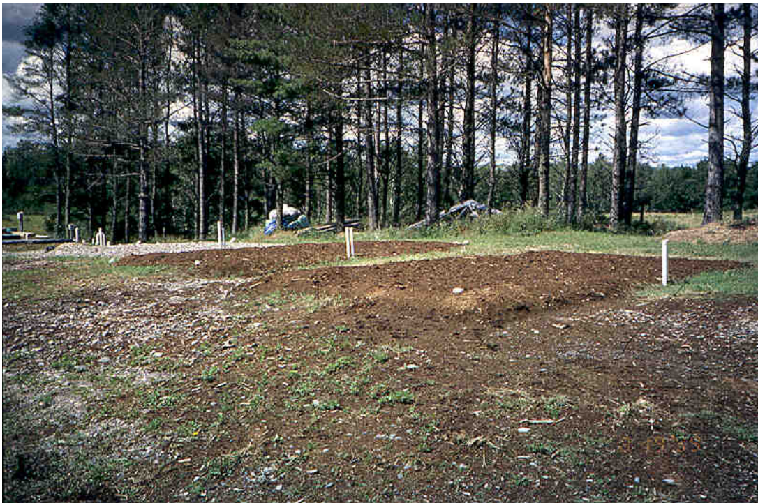
Figure 8. Image of the completed in-ground peat filters.
