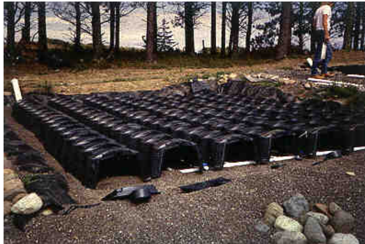
Figure 10. Image of the sand filter chamber covers over the distribution network.
