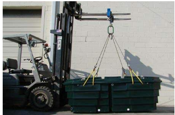
Figure 2 Module Off-loading
