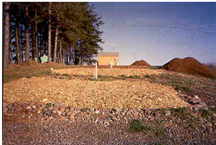
Figure 11. Image of the finished sand filters with the wood chip layer.
