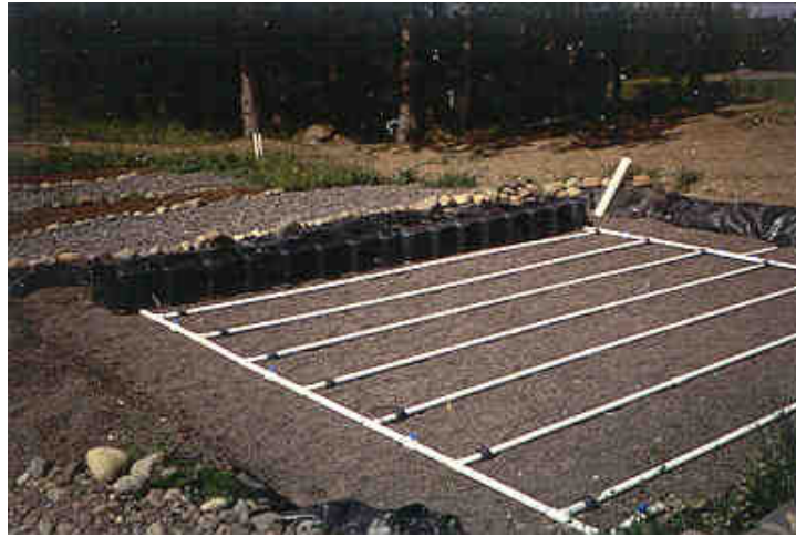
Figure 10. Image of the sand filter chamber covers over the distribution network.
