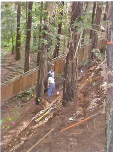
A steep slope installation in California — 65% slope.
