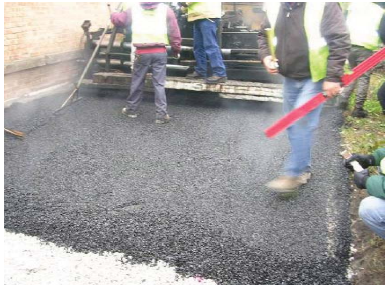
Figure 9: Permeable Asphalt Installation Using Ground Tire Rubber.
