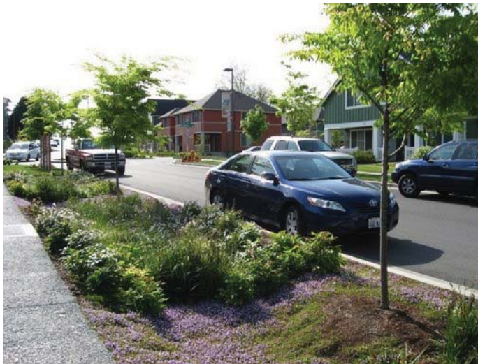
Figure 1. The street-side swale and adjacent porous concrete sidewalk are located in the High Point neighborhood of Seattle, WA (Source: Abby Hall, US EPA).
