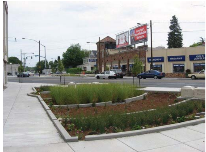
Figure 2. This bioretention area takes runoff from the street through a trench drain in the sidewalk as well as runoff from the sidewalk through curb cuts
